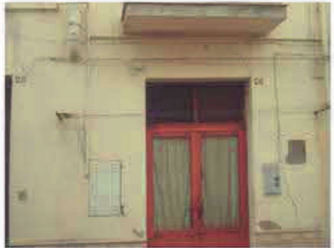
building (8): masonry structure
