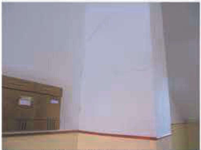
building (13): R.C. structure
