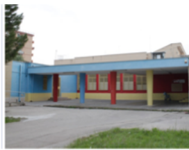
School building “Lopopolo”
