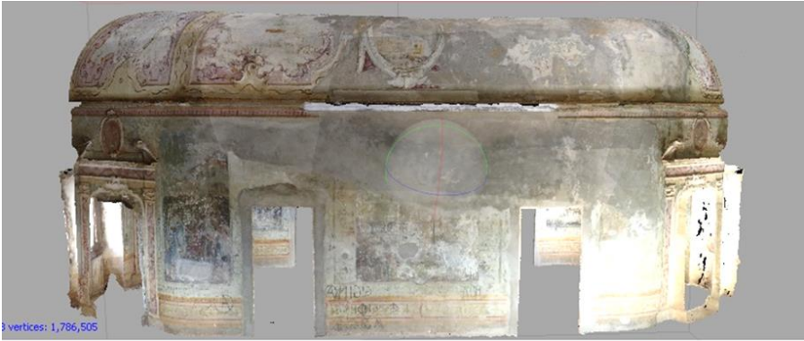
Figure 4.4-4 3D photo-reconstruction in Agisoft Photoscan. Source: author.
