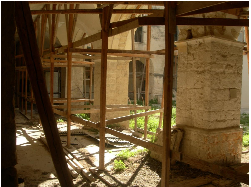
Figure 5.2-2 S.Agostino Monastery: scaffoldings.
