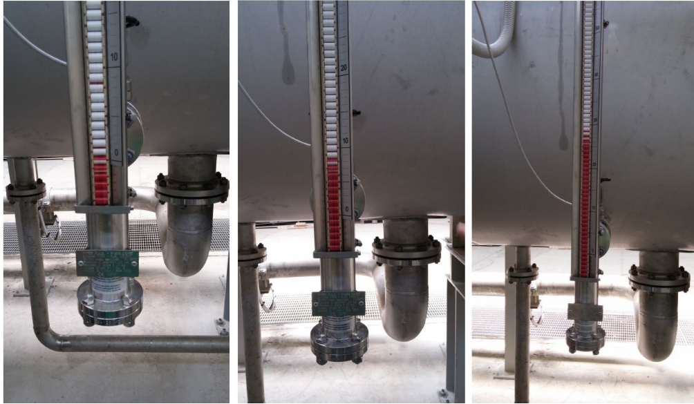
FIGURE 3.4: Magnetic water level indicator during tank filling procedure.
