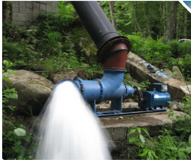
FIGURE 2.3: Example of an axial PAT for rural electrification [27].
