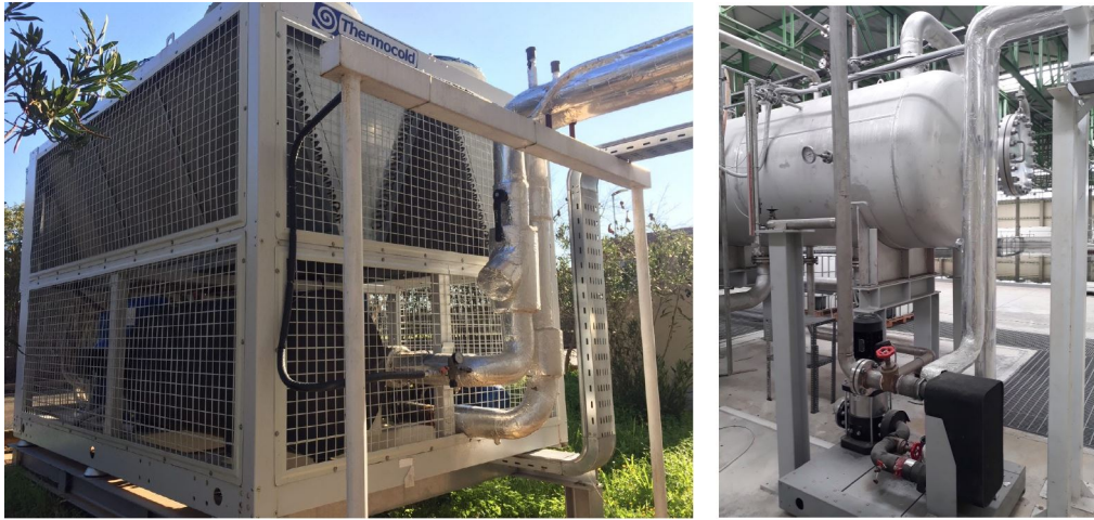
FIGURE 3.5: The Chiller unit (left) and the circulation pump of the cooling system (right).
