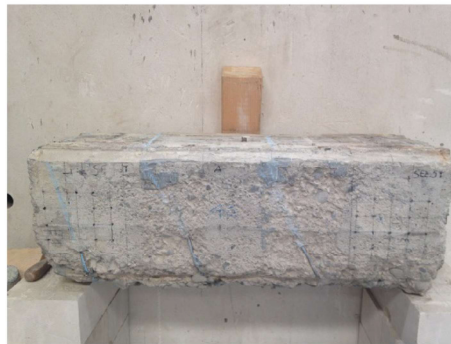
FIGURE 3.20: The intermediate portion of column - floor II
