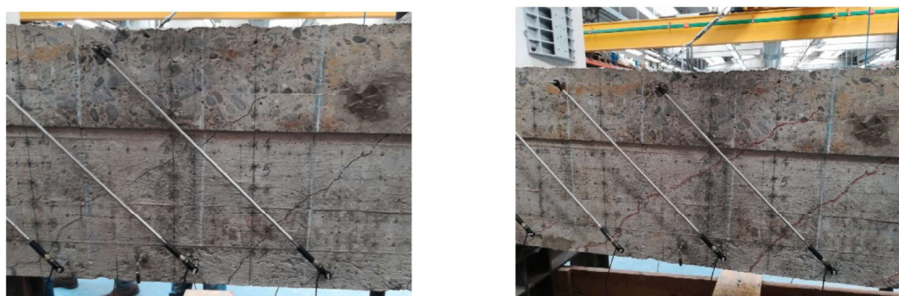
FIGURE 3.92: Shear cracks measured by diagonal potentiometers
