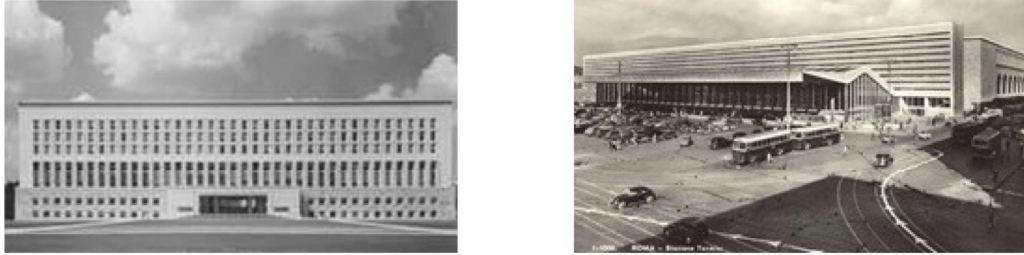
FIGURE 1.29: On left side, Farnesina Building (1937-59); on right side, Termini Railway Station (1939-47)
