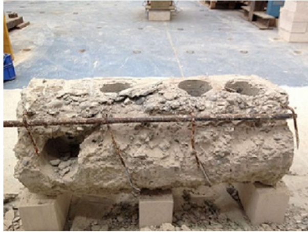
FIGURE 3.25: Extraction steel reinforcement by means of pneumatic drill
