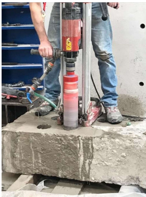
FIGURE 3.1: Concrete cores extraction
