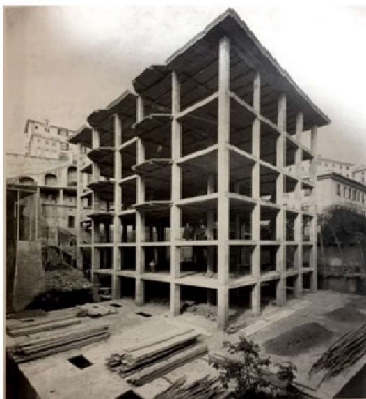
FIGURE 1.4: The first frame house made completely of reinforced concrete and realized by Porcheddu company in Genova in 1906
