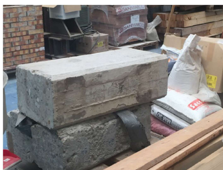
FIGURE 3.17: The top portion of column - floor I
