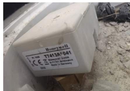
Figure 7: Honeywell - T7413A1041 - Immersion Temperature Sensor. Apolonio Morales 29, Madrid, Control System. Source: Self-elaboration.
