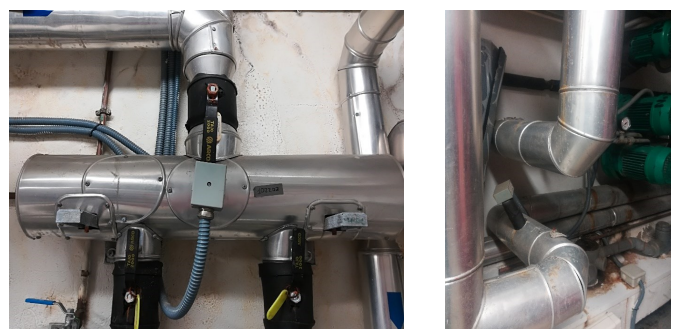
Figure 9: MAMAC SYSTEMS - TE-703-B-17-B-2 - Pipe Temperature Sensors. Apolonio Morales 29, Madrid, Control System. Source: Self-elaboration.
