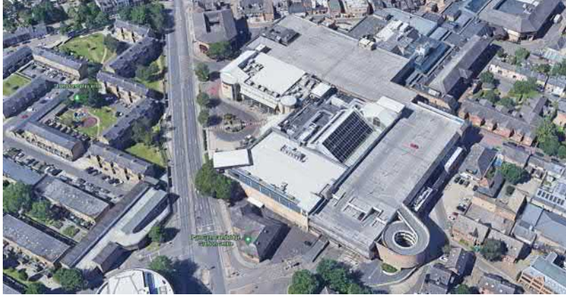
Figure 3.3: Overview of the Grafton East car park, Cambridge (UK) [41].
