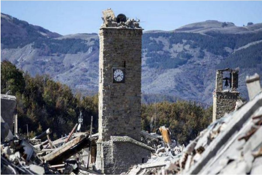
Fig. 1. 4 – Collapse of the Sant'Agostino Bell Tower of Amatrice (Italy) after the 2016-2017 Central Italy earthquake sequence.
