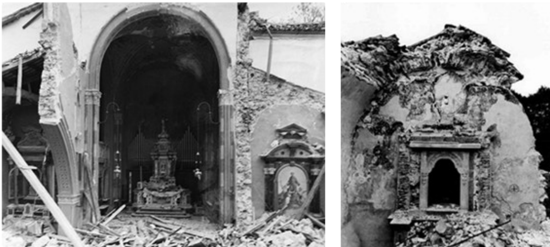
Figure 1: Santa Maria ad Nives Church in Osoppo (left), Ognissanti di Ospedaletto Church in Gemona (right) after Friuli earthquake of 1976.
