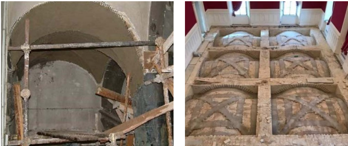
Figure 18: Some examples of strengthening intervention with FRCM [11].
