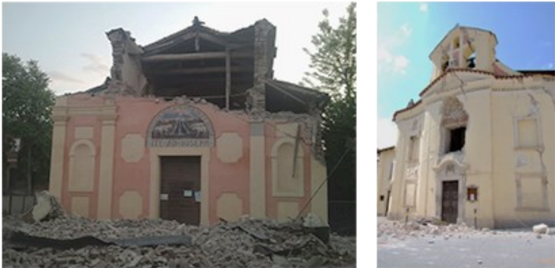
Figure 2: Mulino church in San Felice, after the 2012 earthquake and St. Maria Church in Paganica, damaged by 2009 L'Aquila earthquake.
