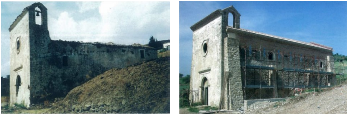
Figure 11: The inclusion of buttresses in renovation intervention, Madonna della Pietà church, Irsina (Matera) [39].
