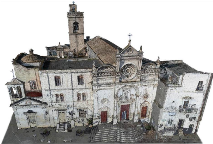
Fig. 22 Integrated point cloud: internal view (on the top) and external view (on the bottom).
