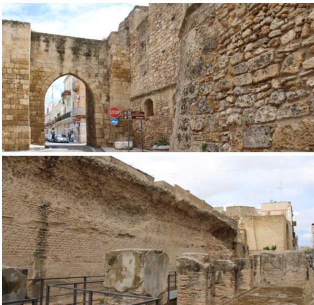
Fig. 8: Remains of the fortified defensive circle of the city of Brindisi. Porta Mesagne and Bastione Carlo (a); walls of Brindisi behind the Piscine Limarie (b) (photos by Chiarello G., Ferrante A., Lamorgese R., Liddo G., Strippoli F., 2022)
