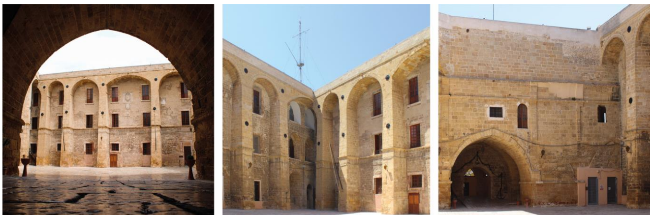
Fig. 12: The Great Castle of Brindisi. Access arch to Piazza d'Armi with northern façade on the back (a), North-Western façade of the Piazza d'Armi (b) south-east façade of the Piazza d'Armi with access arch (c) (photos by Chiarello G., Ferrante A., Lamorgese R., Liddo G., Strippoli F., 2022)
