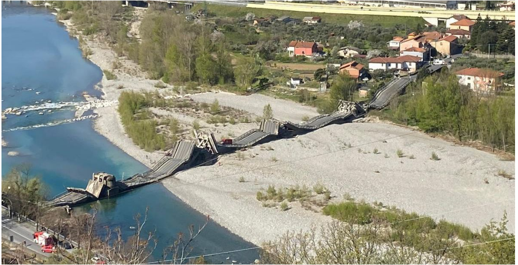
Figure 4 - Albiano Magra bridge collapse.
