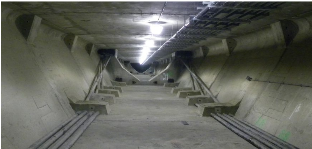
Fig. 75 - Inside view of typical box-girder bridge (Ledesma and WSP USA, 2019).
