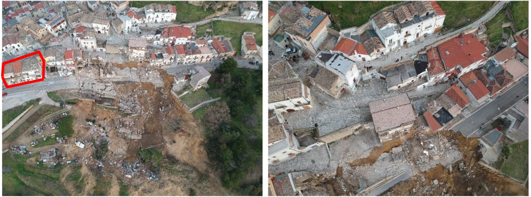
Fig. 62 - Areal views of the Pomarico landslide (left) and focus on damaged structures and infrastructures (right). The red polygon indicates the focused structures.
