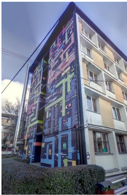
View of the dormitory building
