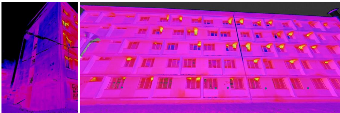
Figure 16. Results for TLS thermal scan for C8 (north and east façade).
