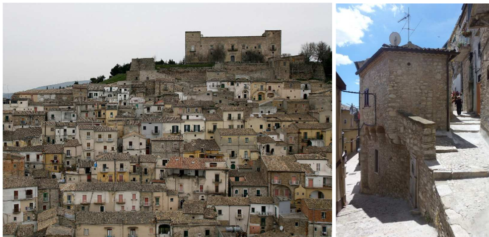
Figure 6: A view of Sant'Agata historical centre (left), and an example of the typical structural aggregate, built on a slope with two level elevations (right).
