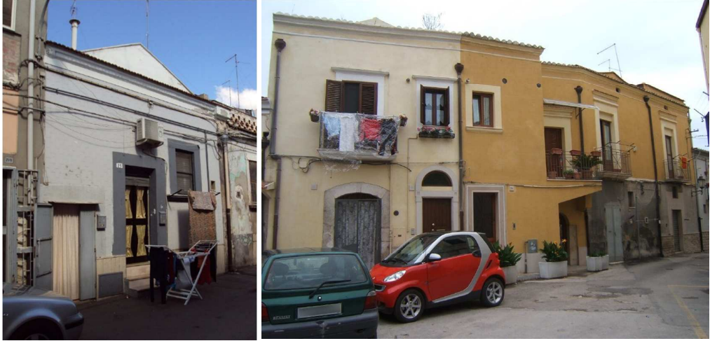
Figure 4: On the left, an example of the original configuration of the houses built after the 1731 earthquake. On the right, the same typology of houses after the addition of a storey and an enlargement.
