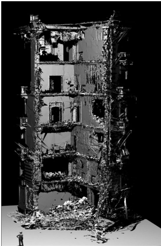
FIG. 7—3D model of collapsed corner.
