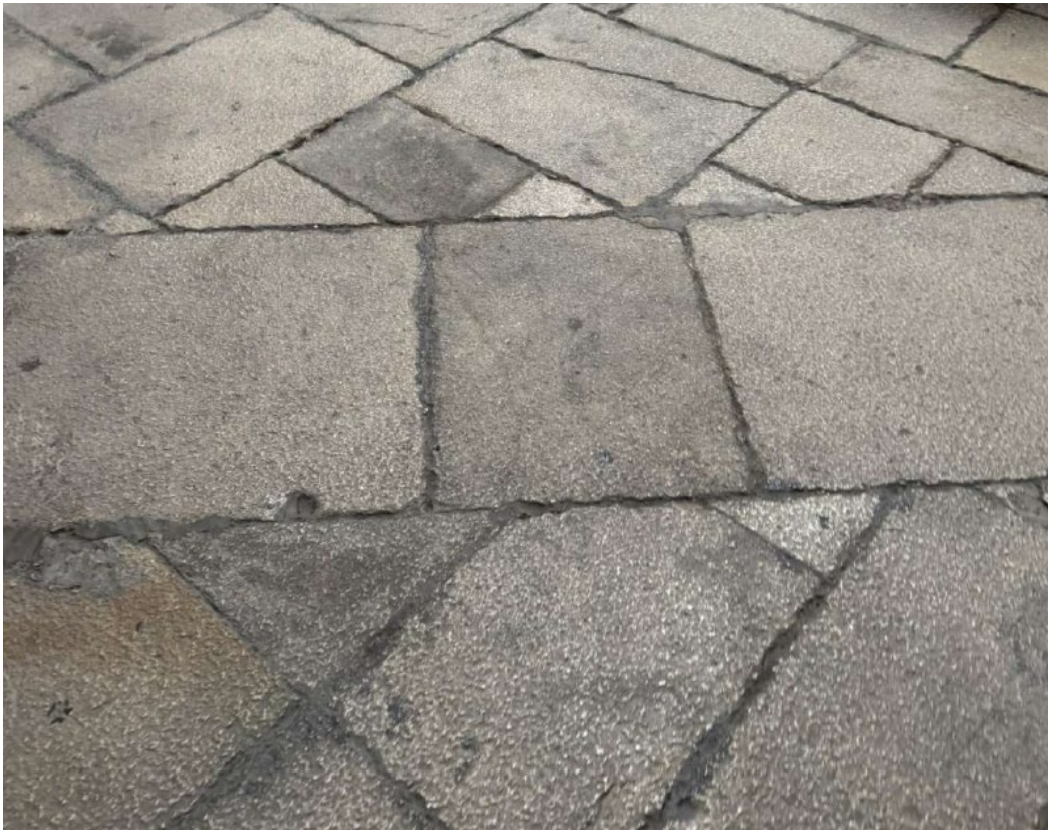
Figure 46 - Paving in local limestone slabs (chianche)
