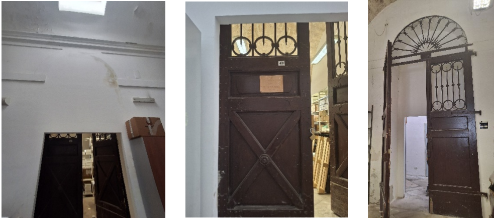
Figure 48 – Drywall partition with opening for access to the space and wooden doorway
