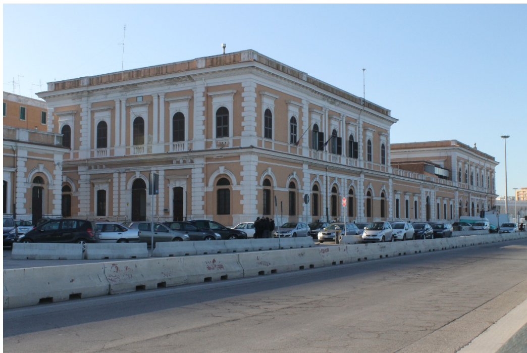
Figure 42 - View from the port area of Palazzo della Dogana
