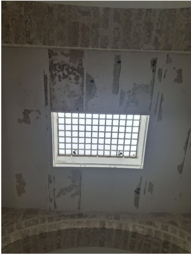
Figure 45 - Rooflights in internal distribution space
