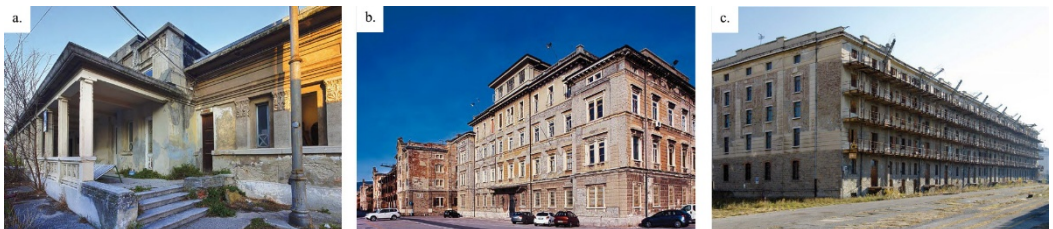
Figure 19 - Assets currently not in use and in a very poor state of conservation: a. Former inn 116, b. Former administration building 118, c. Warehouse 2. Source (Il Porto Vecchio Di Trieste, n.d.)
