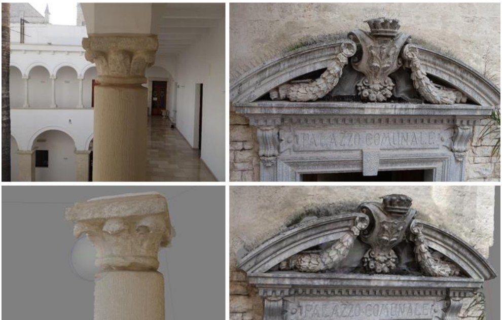
Fig. 33 Textured meshes of the capitals (left) and entrance portal decoration (right) extracted from CRP point cloud of Santa Croce, Monastery, Modugno, Italy
