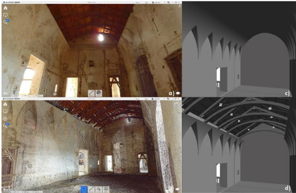
Fig. 93 Internal environment of the building which suffered the collapse of the vault a) and b) point cloud views, c) the old vault, d) the current roof.
