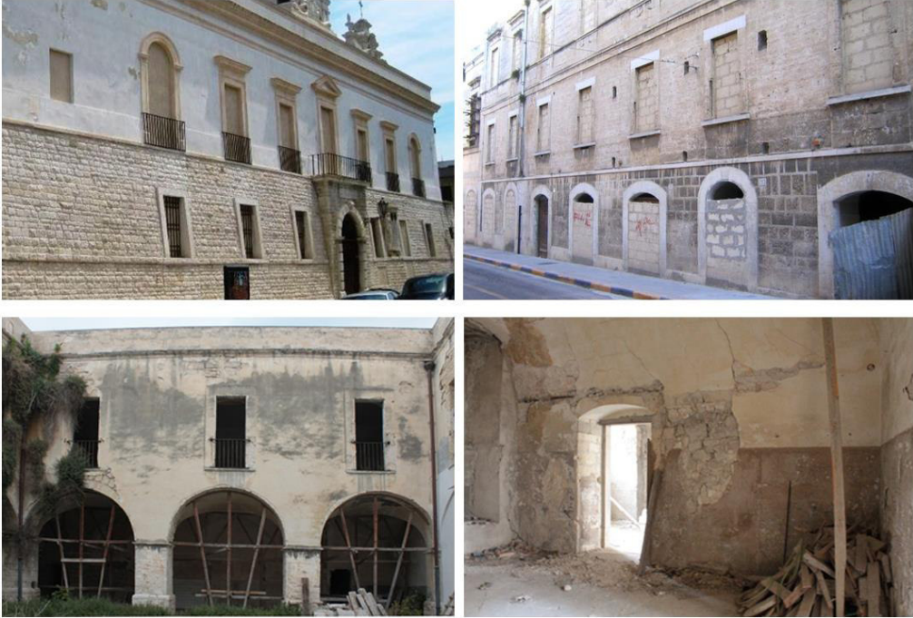
Fig. 78 Photo of the author of Augustinian Monastery: On the top: left, external façade of Unit 1, right, external façade of Unit 2-3, bottom: left, external façade internal cloister, right, a room of Unit 1 on the ground floor.
