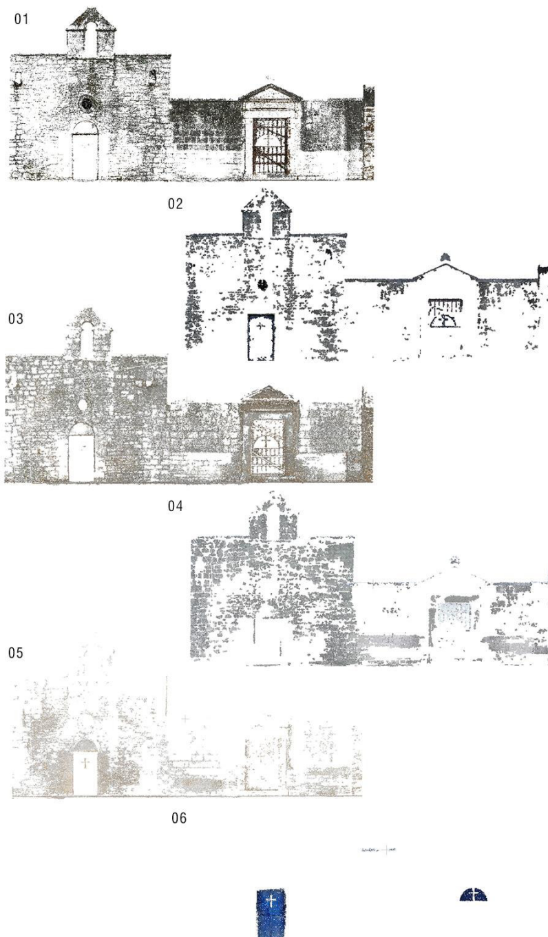
Fig. 55 Clusters in HSV (Case 3-façade Est): 1) biological colonization (46%); 2) spots/deposit (17%);3) moist area (75%); 4) biological patina (67%) 5) unaltered surface (24%);6) doors (7%)
