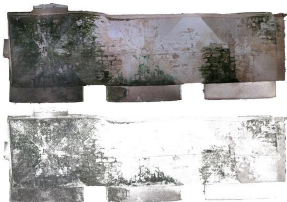
Fig. 46 On the top: Orthophoto of the intrados of the three cross-vaults, below Orthophoto with only green colours extracted
