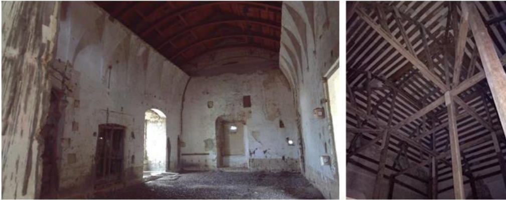
Fig. 76 Current condition of the intervention areas
