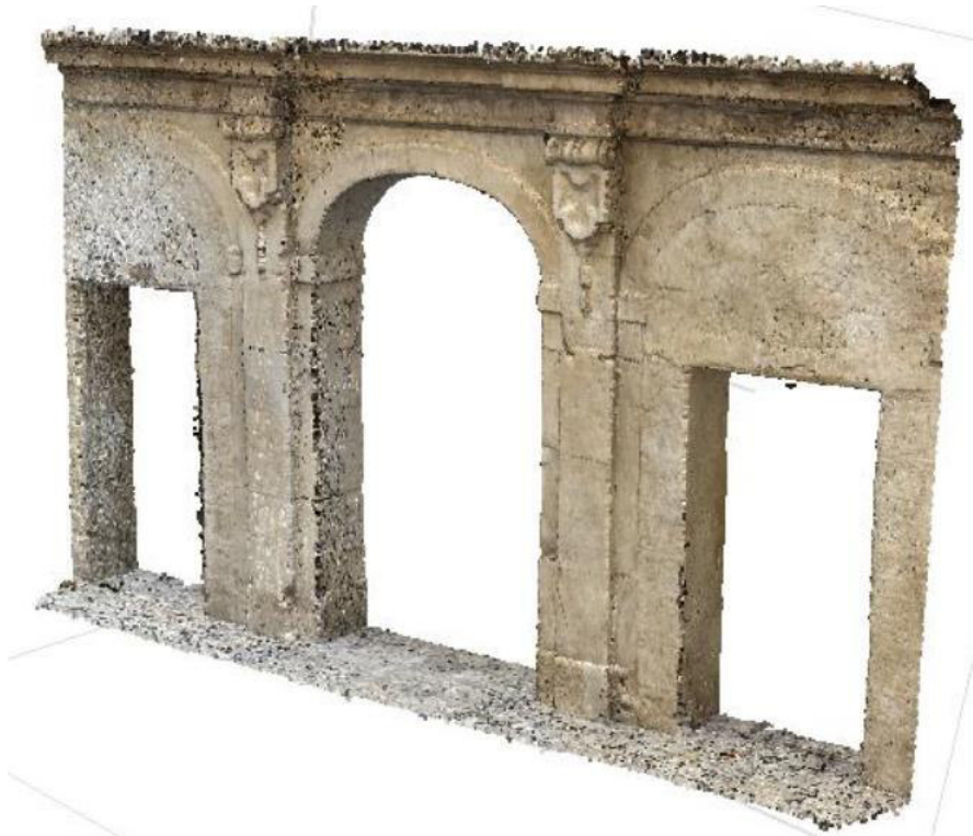
Fig. 2 Example of point cloud of the portal of the inner courtyard of Palmieri Palace, Monopoli (Italy)
