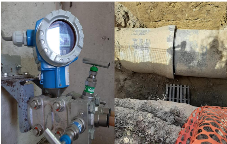
Fig. 6 - The flow meter and irrigation pipeline in pressurized irrigation system at District N. 10.
