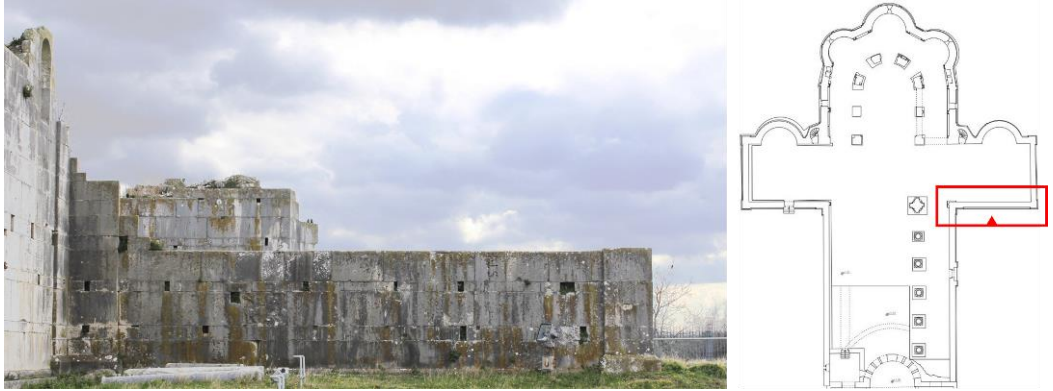
Fig. 51 Southwest façade of the Unfinished Church.
