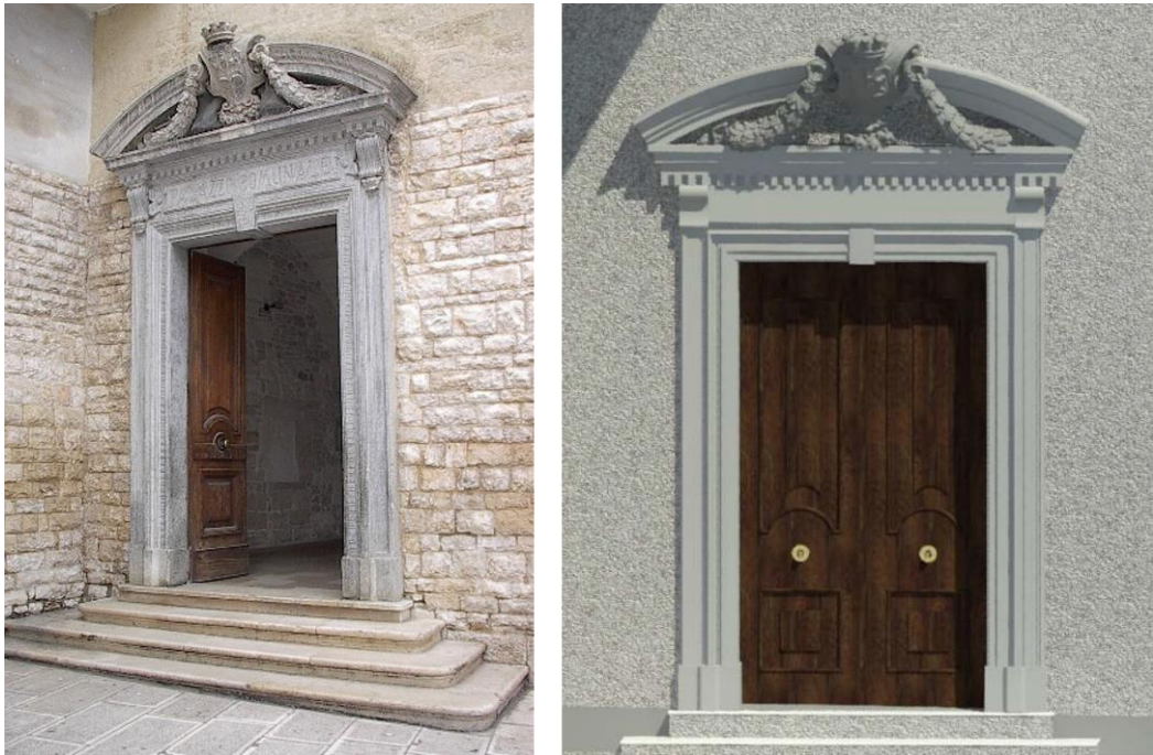
Fig. 36 Entrance portal of the monastery: picture (on the left); parametric family built on Revit (on the right).
