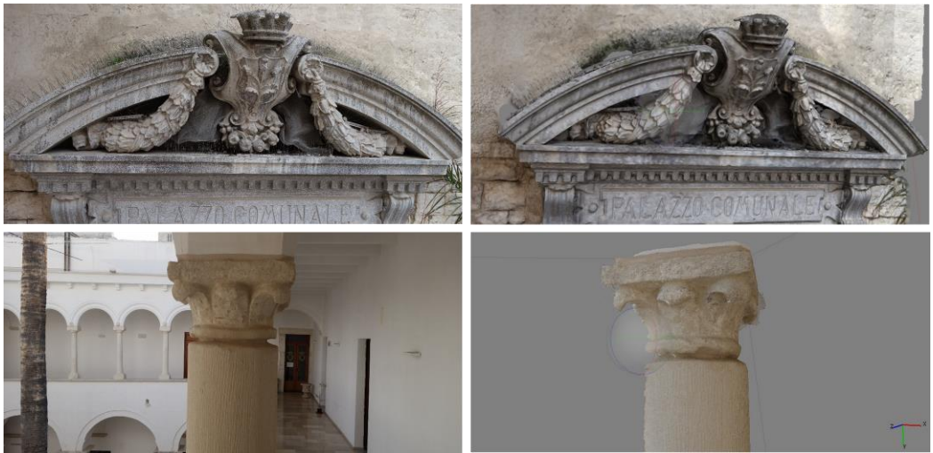
Fig. 35 Pictures of a portal decoration and a capital (on the left); related polygonal meshes (on the right).
