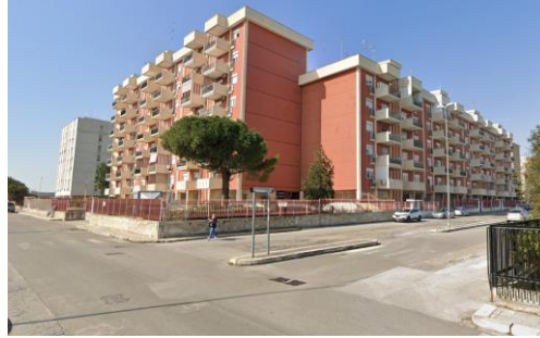
Fig. 4. External view of case study residential buildings cluster.
