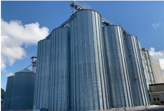
Figure 1-1 View of silos battery used for grain storage with capacity of 3955 tons (Campo San Martino, Italy).
