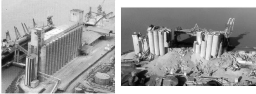
Figure 1-12 Explosion of RC silo Battery (a) before explosion, (b) after explosion, Blaye, France, 1998 (Pineau & Masson, 2001).
