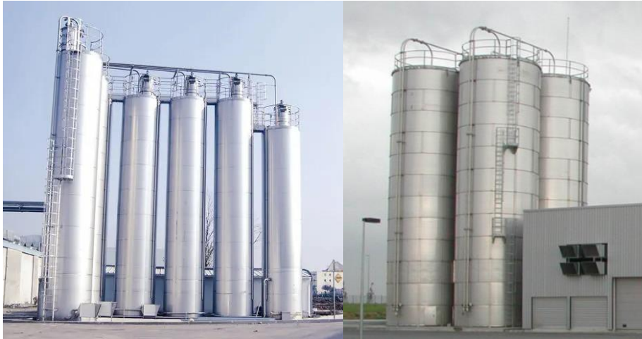
Figure 2-1. Examples of new unstiffened smoothed walls steel silos (from left to right, photos are retrieved from the website of the companies Capi Spa and Technobins, respectively).
