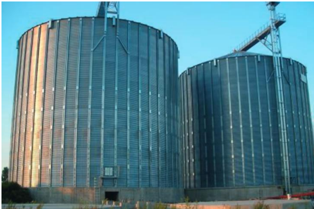
Figure 1-4 Silo corrugated walls in combination with the vertical stiffeners (well-known as silo columns) (Uckan et al., 2015).
