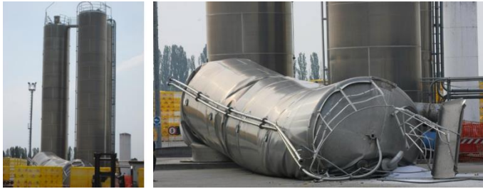
Figure 1-10 Overturning and damages of steel silos due to a seismic swarm hit Emilia Romagna, Italy, 2012 (Butenweg et al., 2017).
