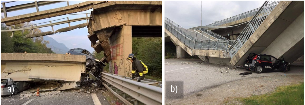
Figure 2 - Annone Viaduct (a), Lecco 2016, and Fossano Viaduct (b), Cuneo 2017
