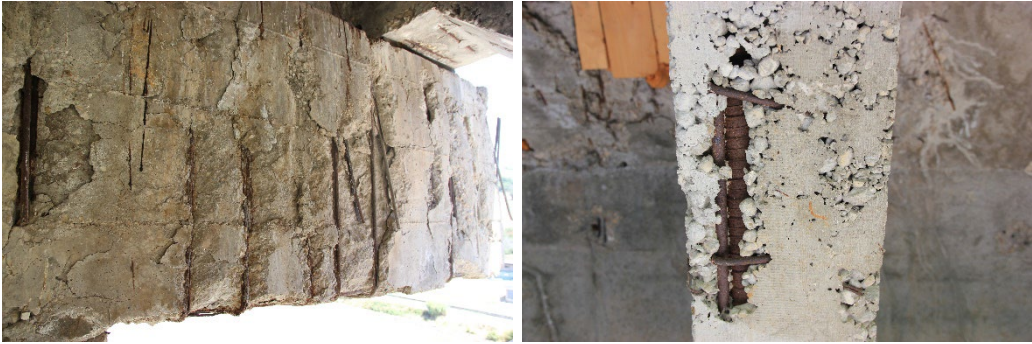
Figure 7 - Degradation of concrete structures.
