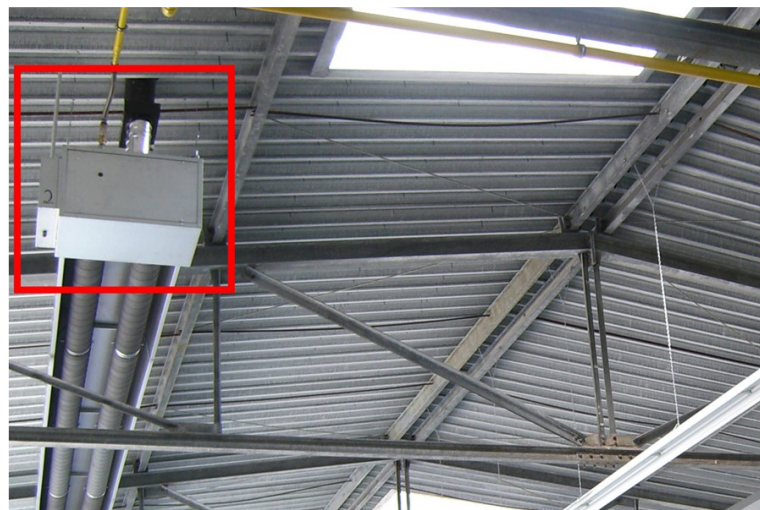
Fig. 39 Example of installation of a gas-fired radiant heating system (in red) on the roof of an industrial warehouse.
