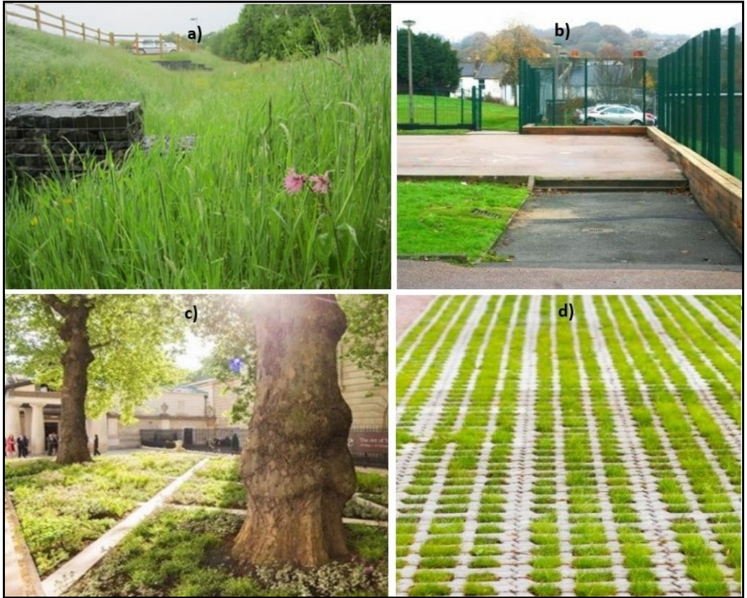
Fig. 2 – Examples of urban BG infrastructure at different scales. a) Wetland in Kington, Herefordshire 3 . b) Swale in Hastings, England 4 . c) Trees in London, England 5 . d) Permeable paving in Oregon, USA 6 .
