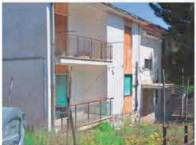
building (26): masonry structure
