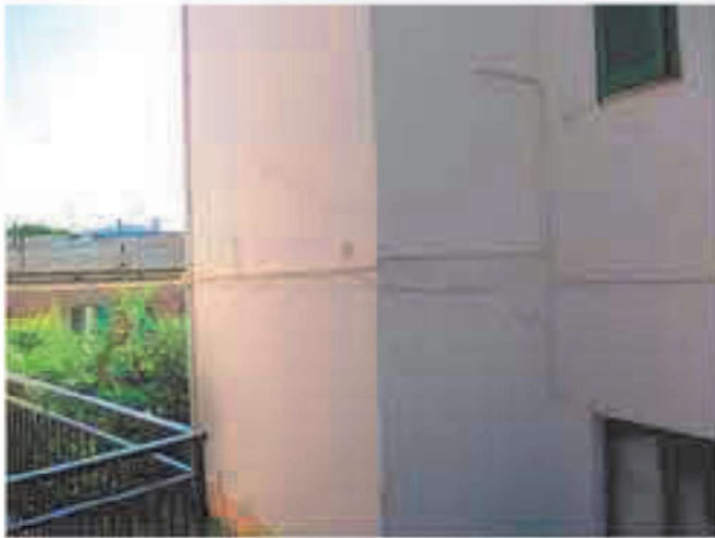
building (6): masonry structure
