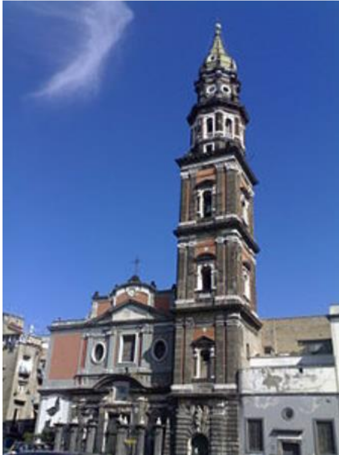
Fig. 2. 21 – View of the Carmine monumental complex located in Naples.
