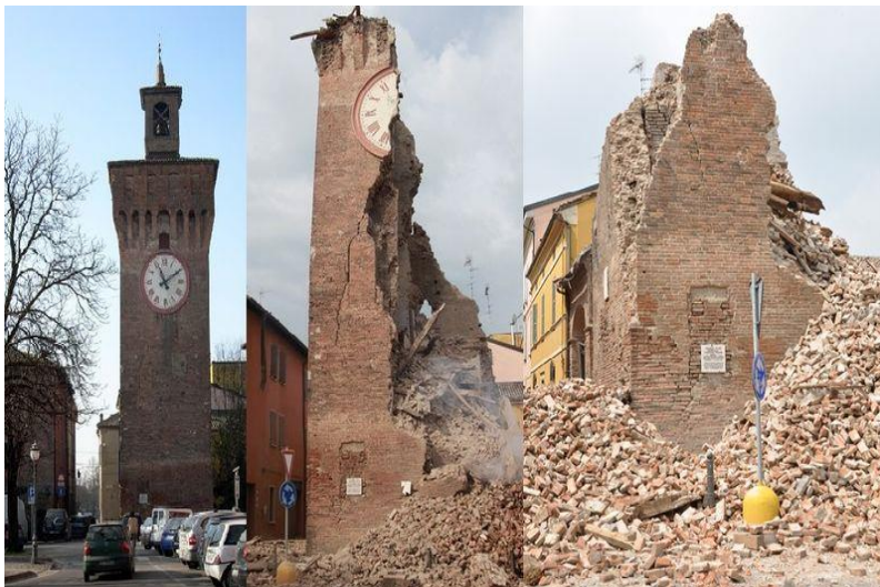
Fig. 1. 3 – Collapse of the Finale Email Clock Tower (Italy) after the May 2012 Emilia Romagna earthquake sequence.
