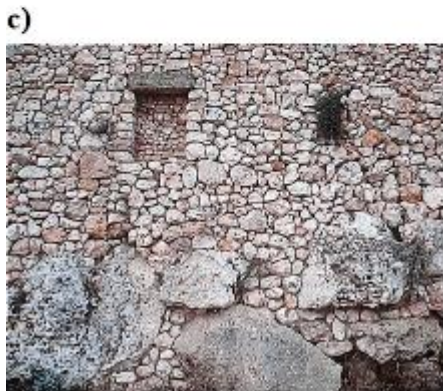
Fig. 3. 4 – Different stone masonry types: a) perfectly regular square units, b) irregular square units, c) rubble and d) dry stack masonry walls.
