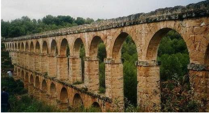
Fig. 3. 2 – Ancient Roman aqueduct Les Ferreres, Tarragona (Spain).
