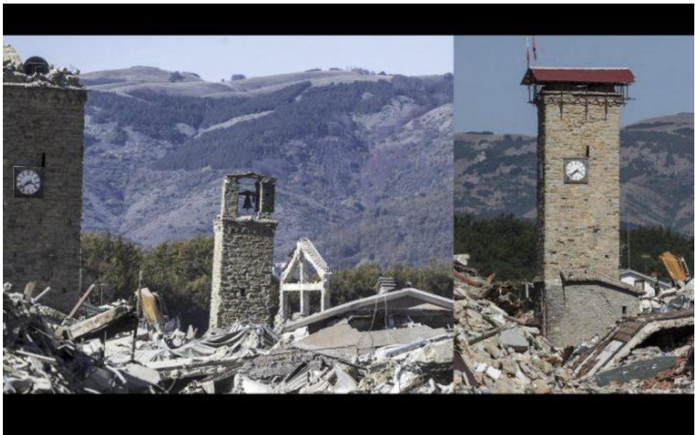
Fig. 2. 20 – Collapse of the Sant'Agostino Bell Tower in Amatrice due to soil amplification effects.
