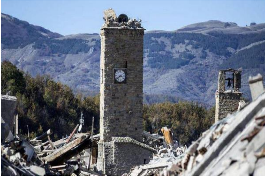
Fig. 1. 4 – Collapse of the Sant'Agostino Bell Tower of Amatrice (Italy) after the 2016-2017 Central Italy earthquake sequence.
