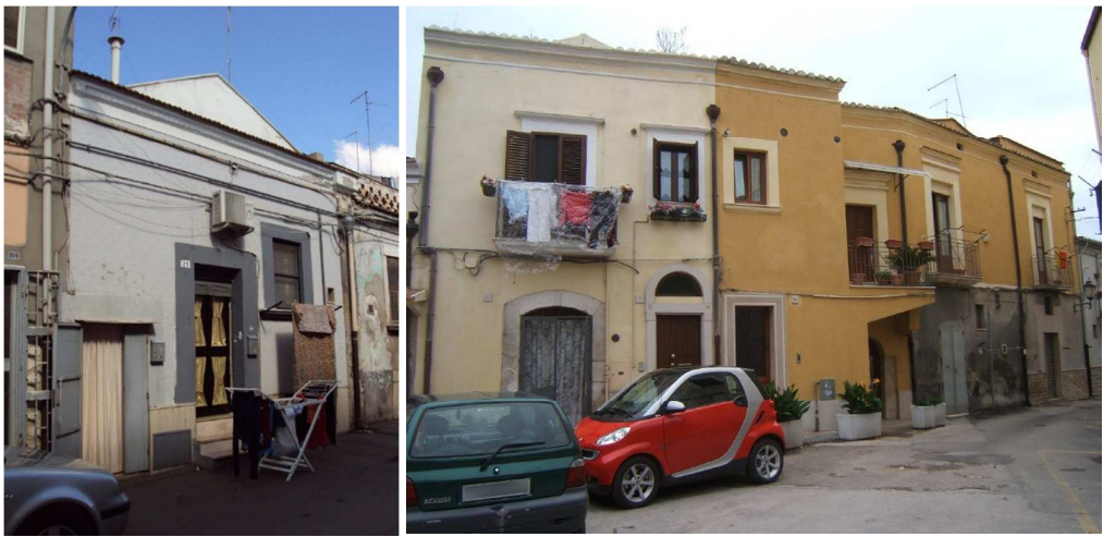
Figure 4: On the left, an example of the original configuration of the houses built after the 1731 earthquake. On the right, the same typology of houses after the addition of a storey and an enlargement.
