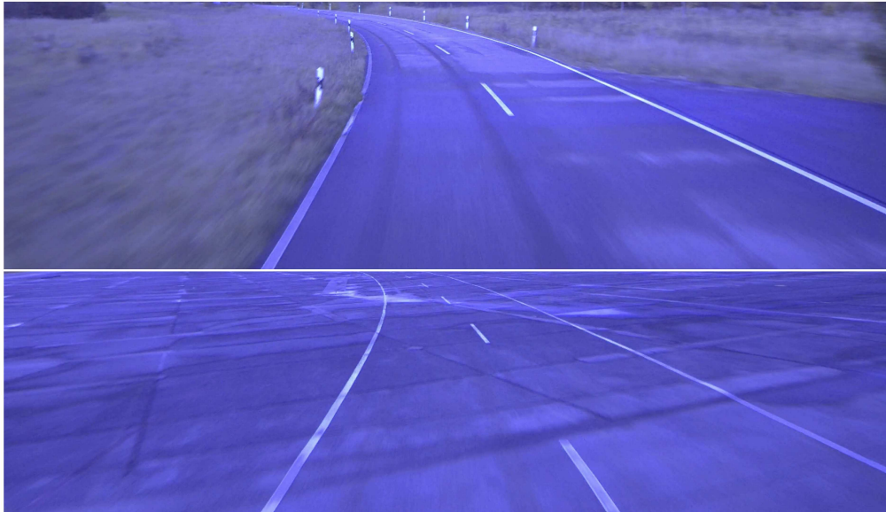
Figure 9.9: Tyre marks (top image) left on the track after multiple laps, which closely overlap along most of the circuit. Discrete road blocks (bottom image) which composed part of the track tarmac.
