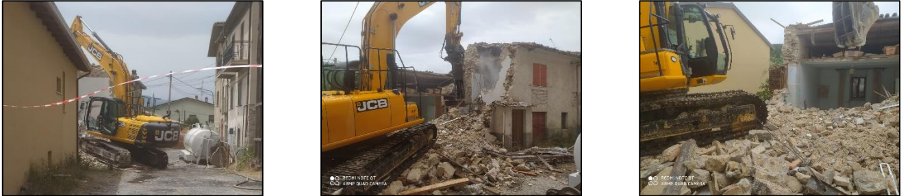
Figure 9. Three different stages of demolition.
