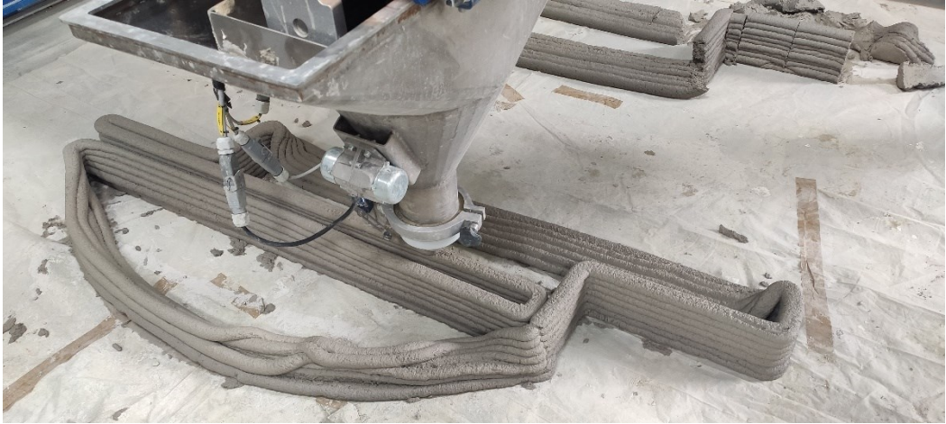
Fig. 39 Example of layers' collapse, probably due to the slenderness of the walls and the breakage of the sloping surface.
