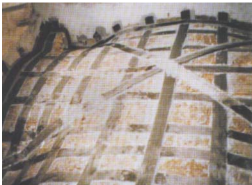
Reinforcements of vaults by FRP
