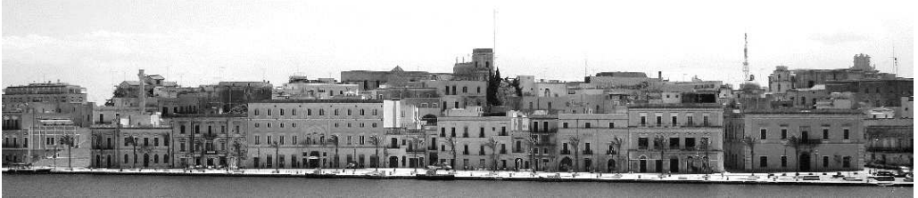
Figure 7. 10 The inner port: historic centre, Roman Columns and promenade R. Margherita
