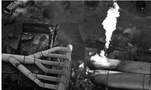
Figure 5.3 Image of a jet fire
