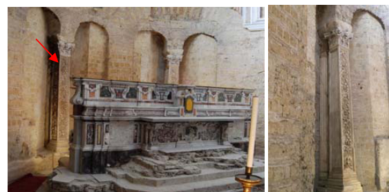
Fig. 1. Monolithic marble columns (II century) in the early Christian apse (VI century) located behind the baroque altar (XVIII century).
