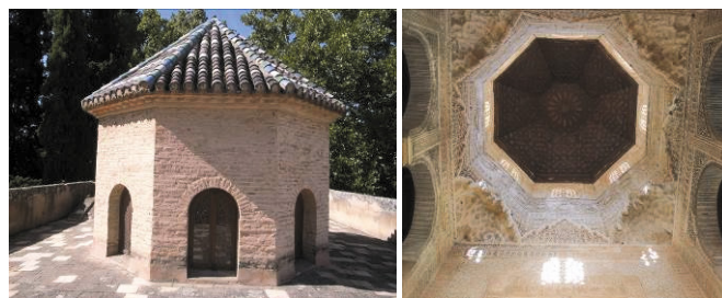
Fig. 2. Views of the lantern outside and inside.
