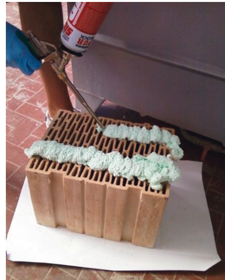
FIGURE 5: Placement of the foam.
