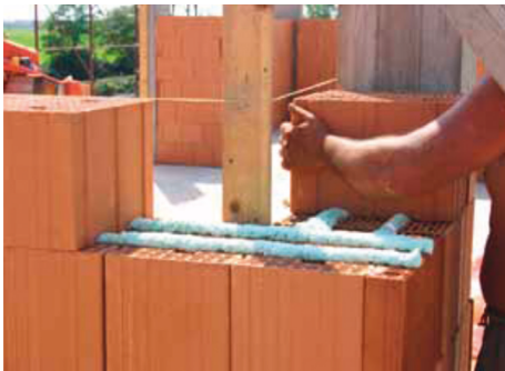
FIGURE 17: Example of foam placement on the brick.
