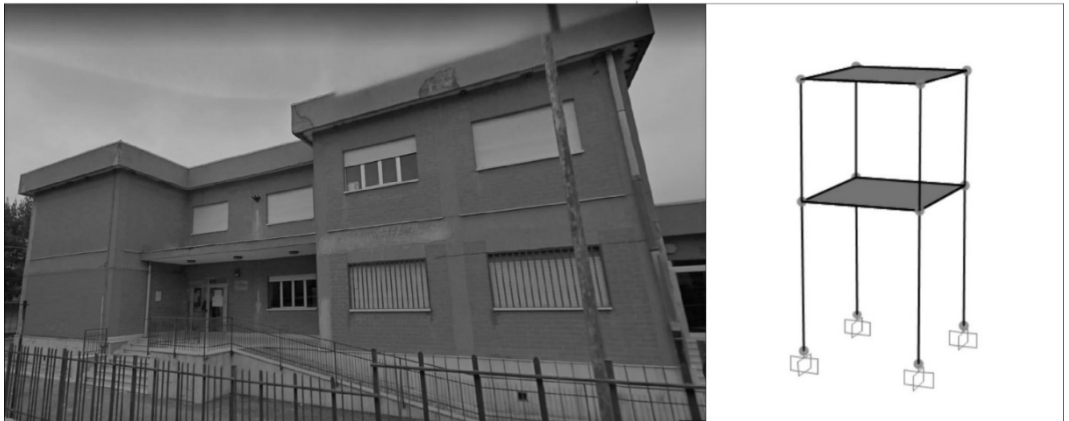
Fig. 5.19 – Concept of our 3D reduced-order model, applied on a case studied (B10)
