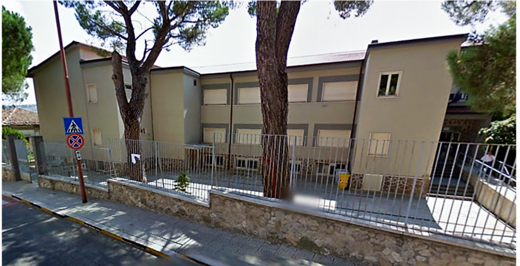
Fig. 4.20 – Picture of the existing RC school building investigated
