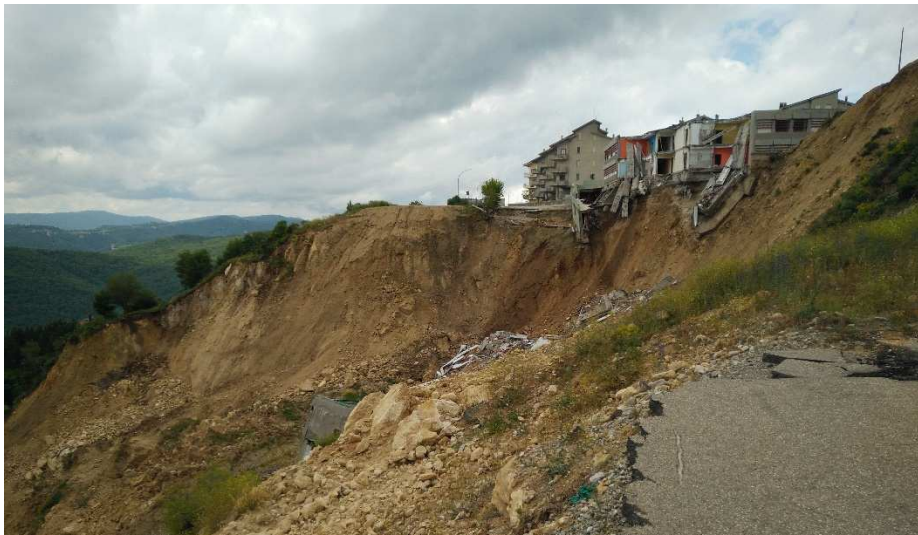
Fig. 18 - The complex landslide of Stigliano municipality (Basilicata region, Southern Italy) that affect buildings and roads within a building expansion area of the '80s.
