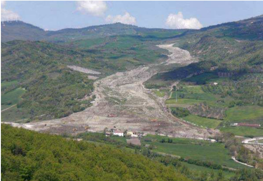
Fig. 17 - Earthflow landslide in Montaguto (Campania region, Southern Italy) that, in 2010, affected the national road SS 90 and the national railroad (source: http://www.irpi.cnr.it ).
