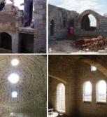
1.Stone excavated from Site re-used for foundation construction 2.Construction of load-bearing walls using block bonding 3.Vaulted ceiling are built using local wooden shutters 4.Fireplace construction 5.North Courtyard 6.South elevation view before closing the walls 7.Hammering the keystone using raw stone 8.Bath Tub Domed ceiling 9.Living area internal view 10.Vaulted ceiling after removing the shutters
