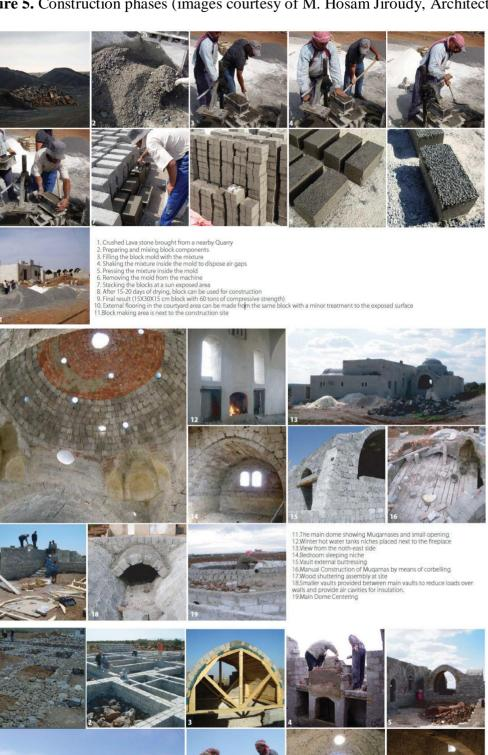
Figure 5. Construction phases (images courtesy of M. Hosam Jiroudy, Architect).
