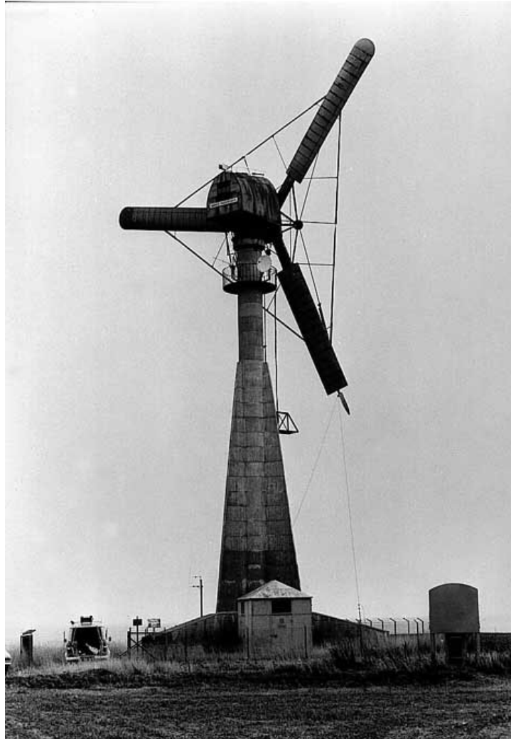
Figure 1.1: The three-bladed wind turbine built by J. Juul in 1957 near Gedser (Zealand, Denmark). Juul's turbine established the so-called "Danish design" which was adopted by manufacturers around the globe as reference for the development of modern wind turbines.
