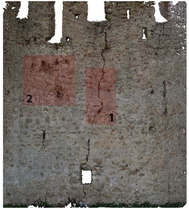
Fig. 3. Point cloud of an extended portion of the north tower (covered area of about 60 m 2 ), with the indication of the two samples (1, 2) used for the application of the methodology.
