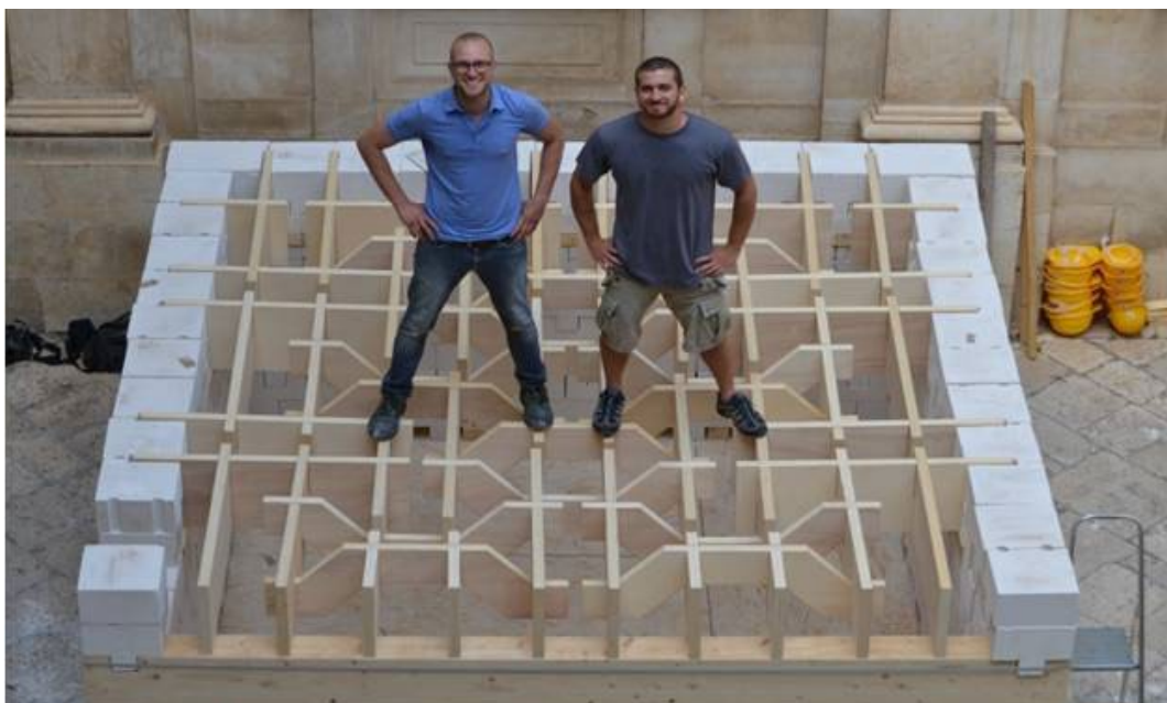
Figure 3. The prototype created during the ‘Self Made Architecture 01’ summer school.
