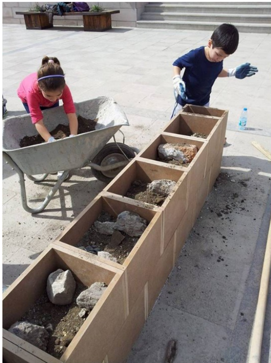
Figure 4. A moment in the construction of the prototype of the ‘Self Made Architecture 02’ summer school.
