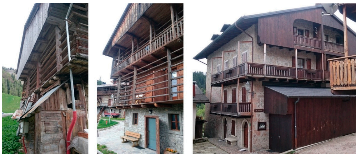
Figure 5. Examples of different load-bearing structural systems in Sauris di Sopra settlement—image taken by the authors.
