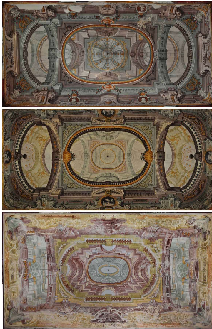
Figure 5. Bottom view by photogrammetric surveys of the vaults of the palaces Broquier in Trani, Manes in Bisceglie and the Baronial palace in Botrugno (V. Castagnolo, G. Rossi).
