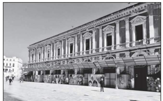
Figure 2 - The former Fish Market building - current state
