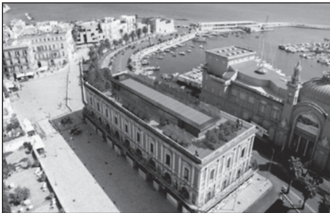
Figure 3 - The former Fish Market - project situation. On the right the Margherita Theater
