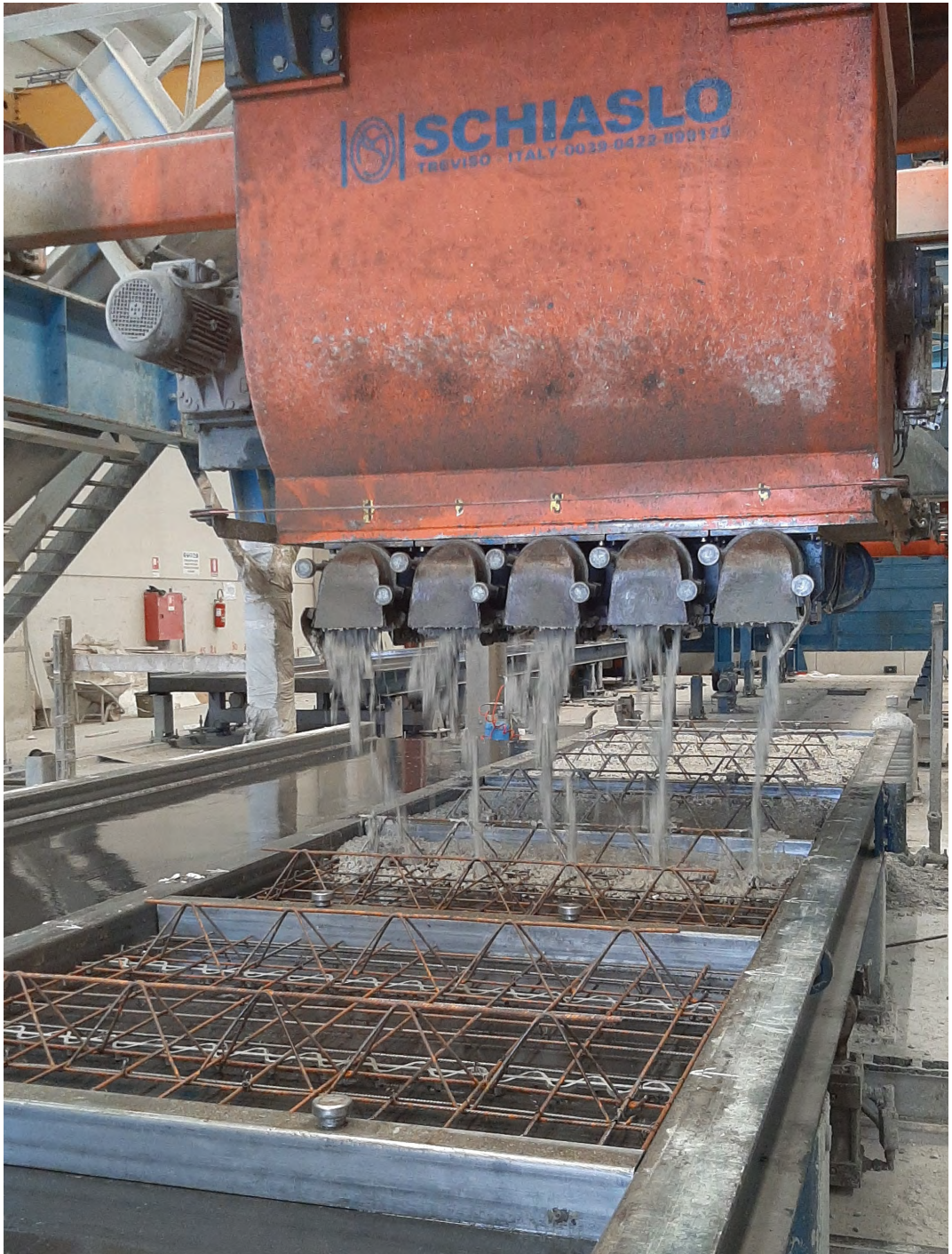
Figure B.10: Concrete casting until the custom thickness
