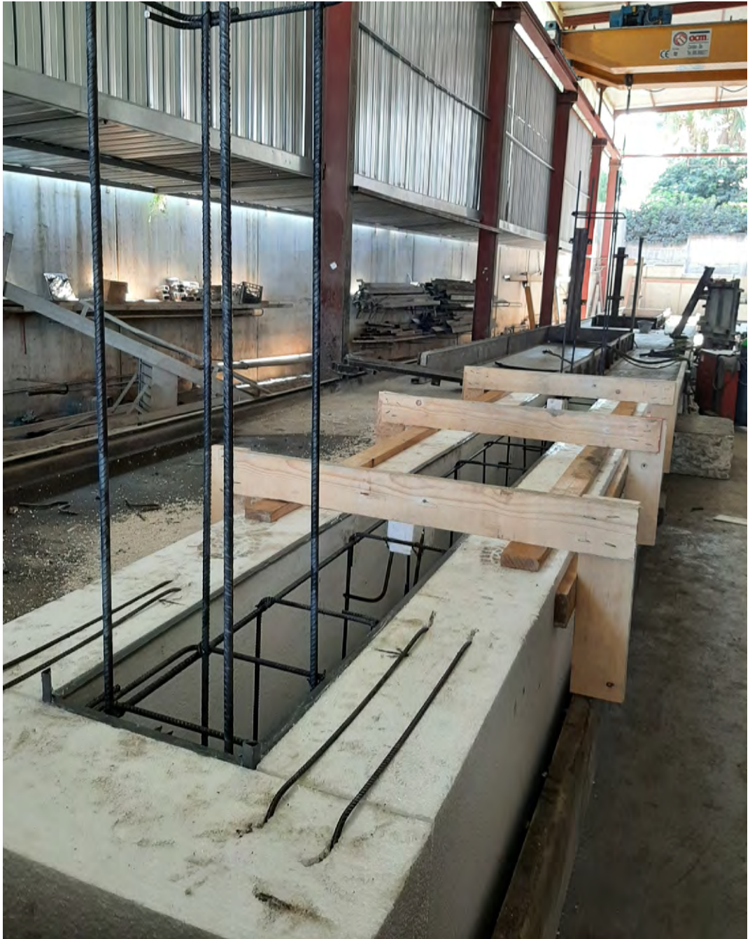
Figure C.1: Wall foundation: construction of the formwork and reinforcement assembling
