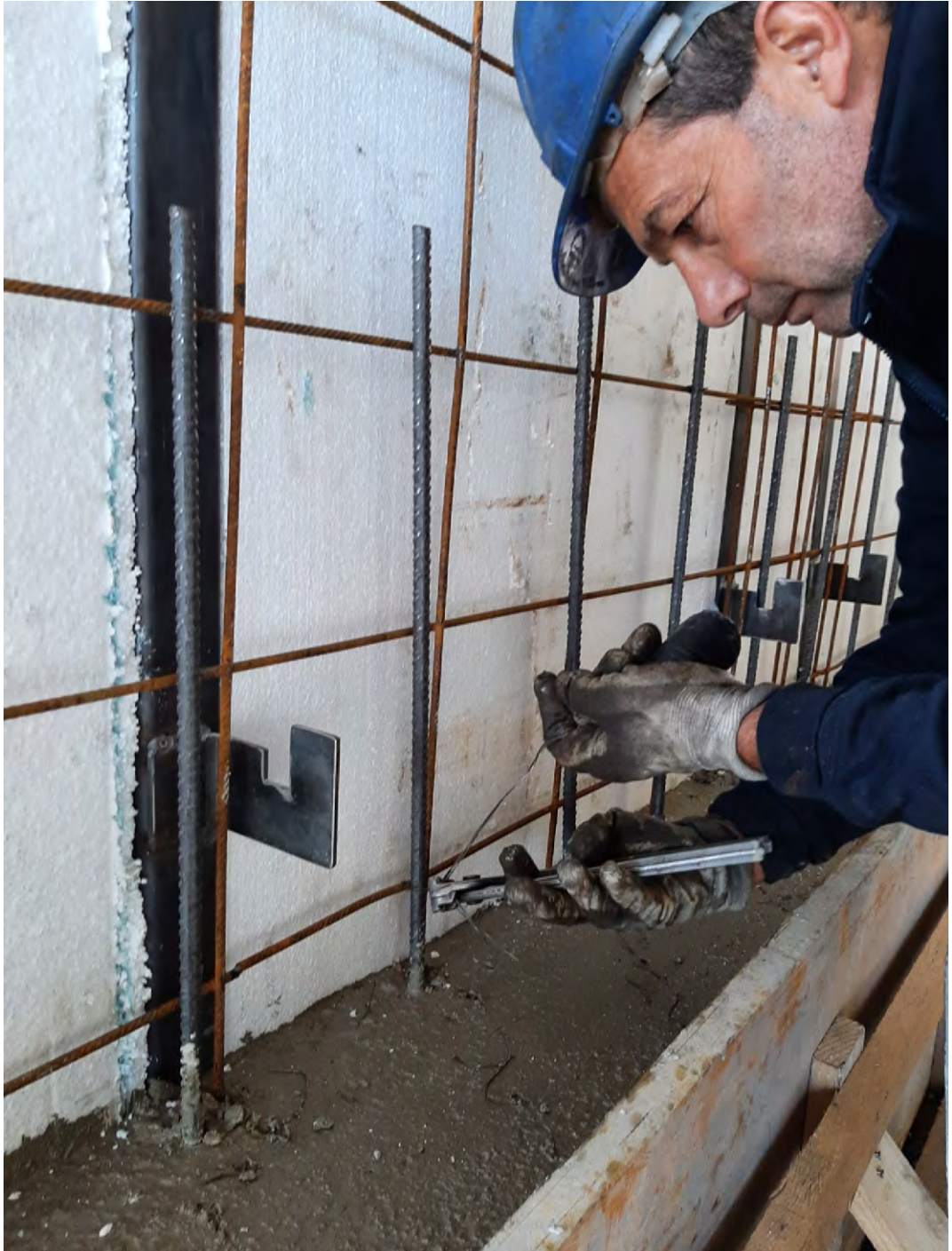
Figure E.23: Binding of the connecting bars with the reinforcement mesh
