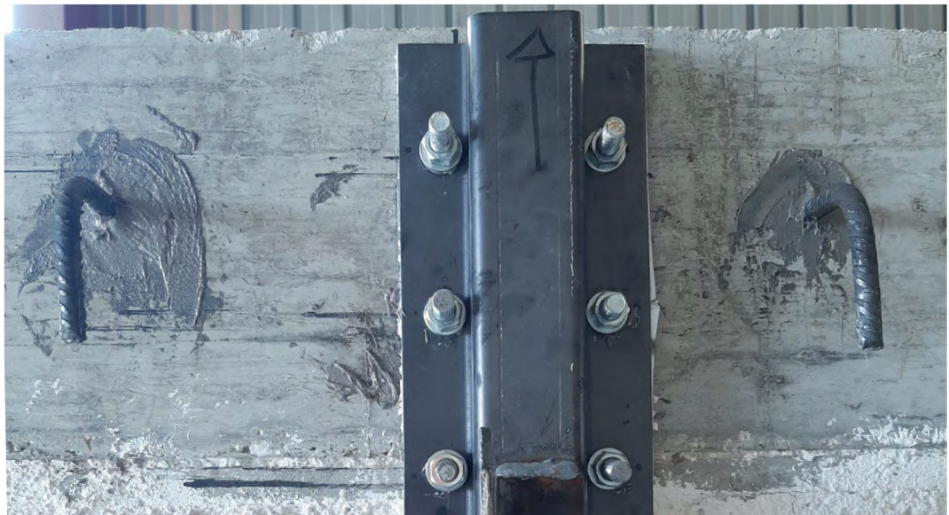
Figure E.10-11-12: Insertion and tightening of washers and bolts
