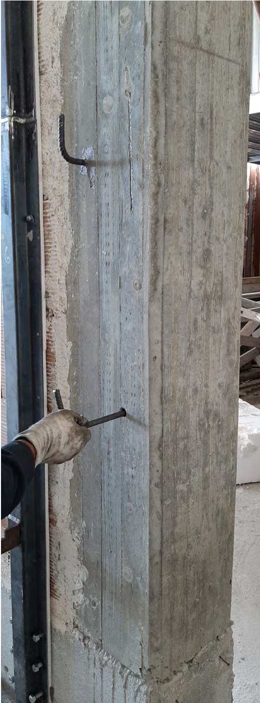
Figure E.7-8-9: Post-installed rebars insertion into the chemical injected holes
