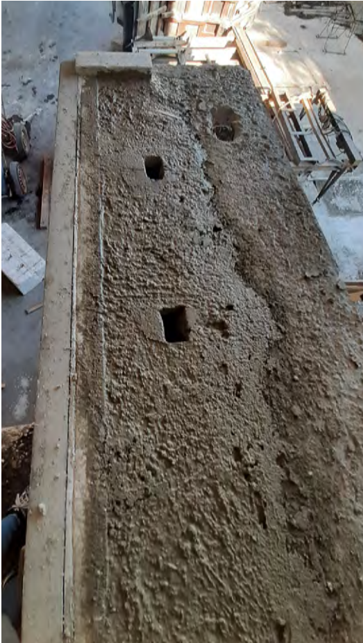
Figure E.50-51: Closing surface of the IPCS after LWSC casting: fresh state (left); dry state (right).
