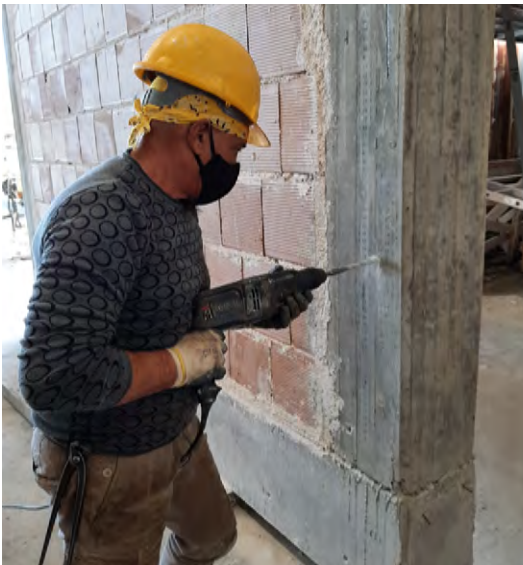
Figure E.1-2-3: Drilling of the concrete frame up to the calculated depth for chemical injection and anchoring of post-installed reinforcing bars and connectors
