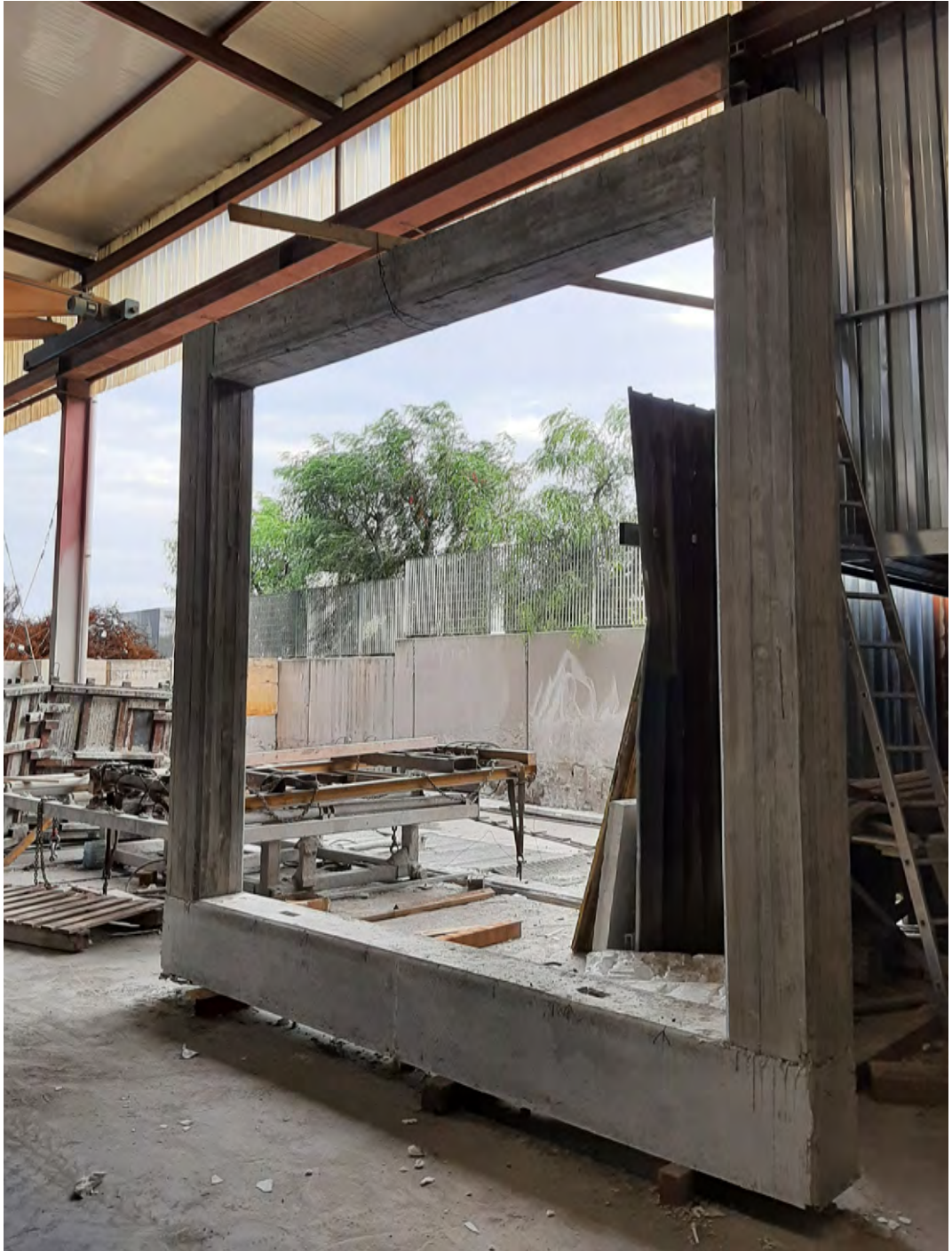
Figure C.3: Concrete frame of the wall sample
