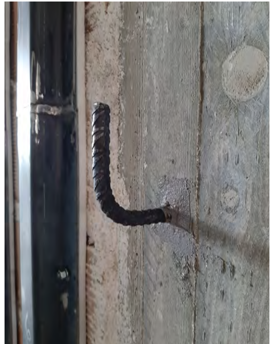
Figure E.7-8-9: Post-installed rebars insertion into the chemical injected holes
