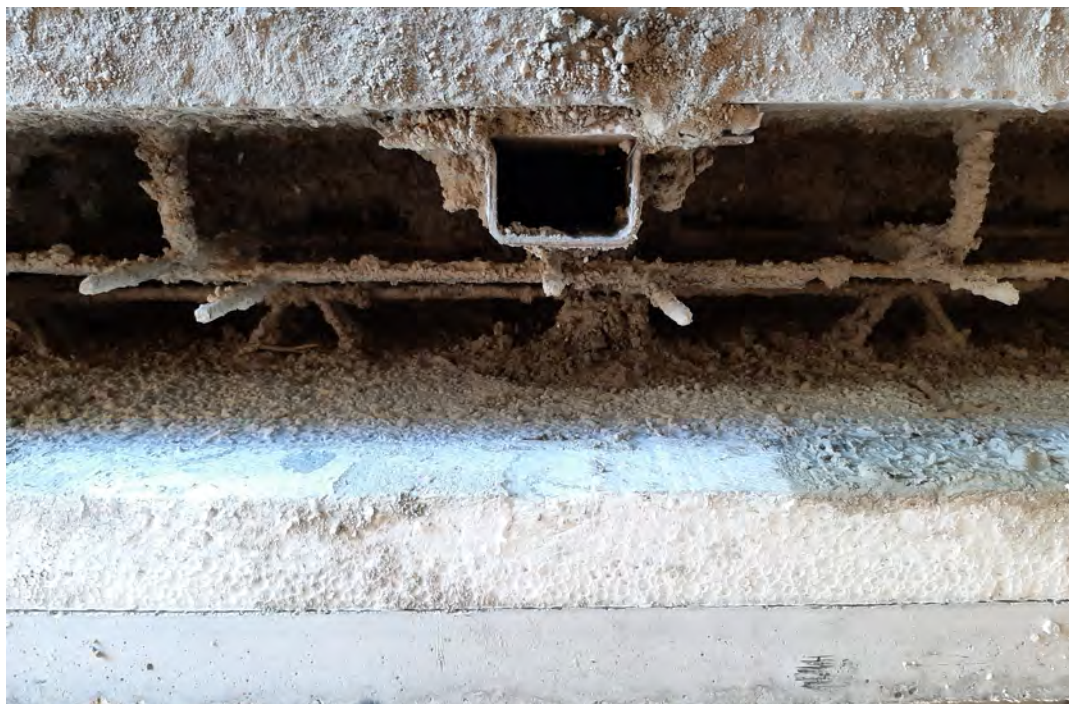
Figure E.43: Detail of the omega profile of the empty mullion (top view)
