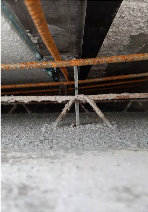
Figure E.38-39: Anchoring details (top view)
