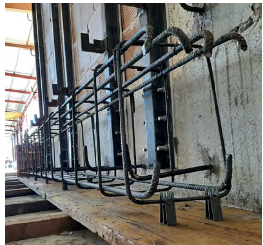
Figure E.15-16-17: Assembling of the foundation rebars of the system
