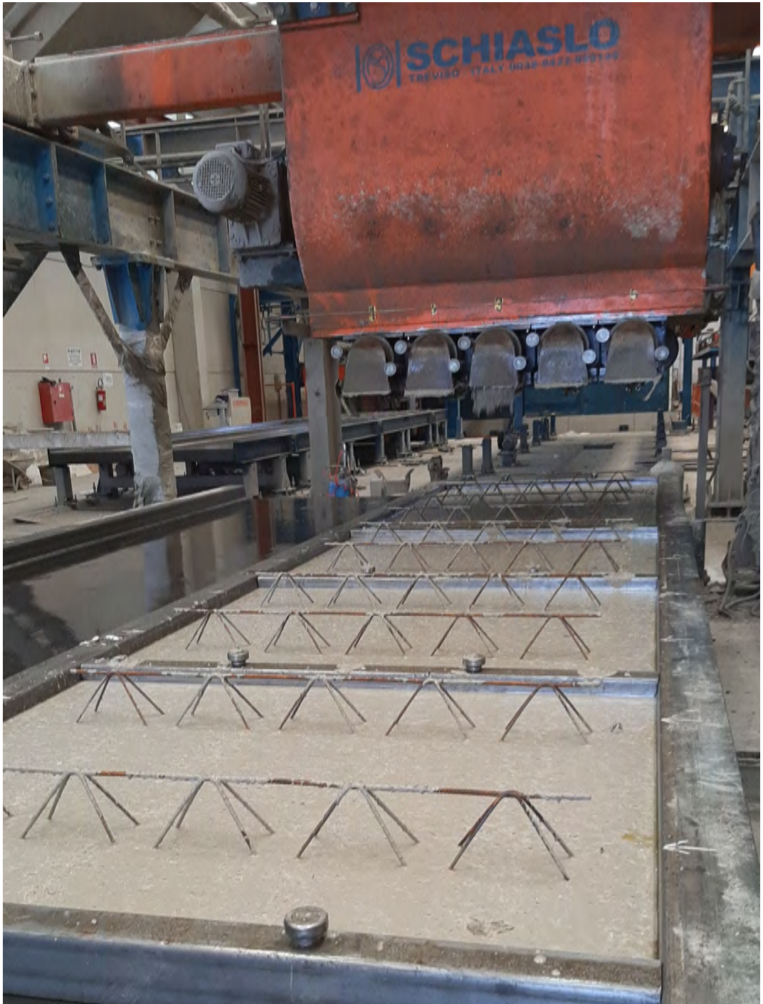
Figure B.13: Mechanical vibration of the formwork
