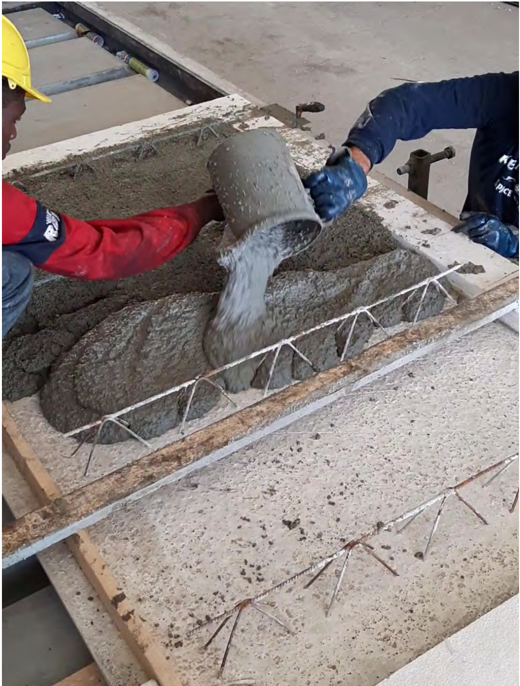
Figure B.20: LWM casting on the inner face of the base modules up to 5 cm
