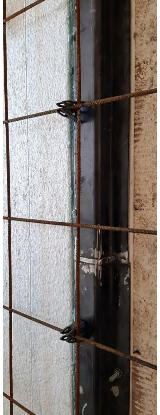
Figure E.26: Insertion of the spacers to assure the concrete cover as the calculating drawings
