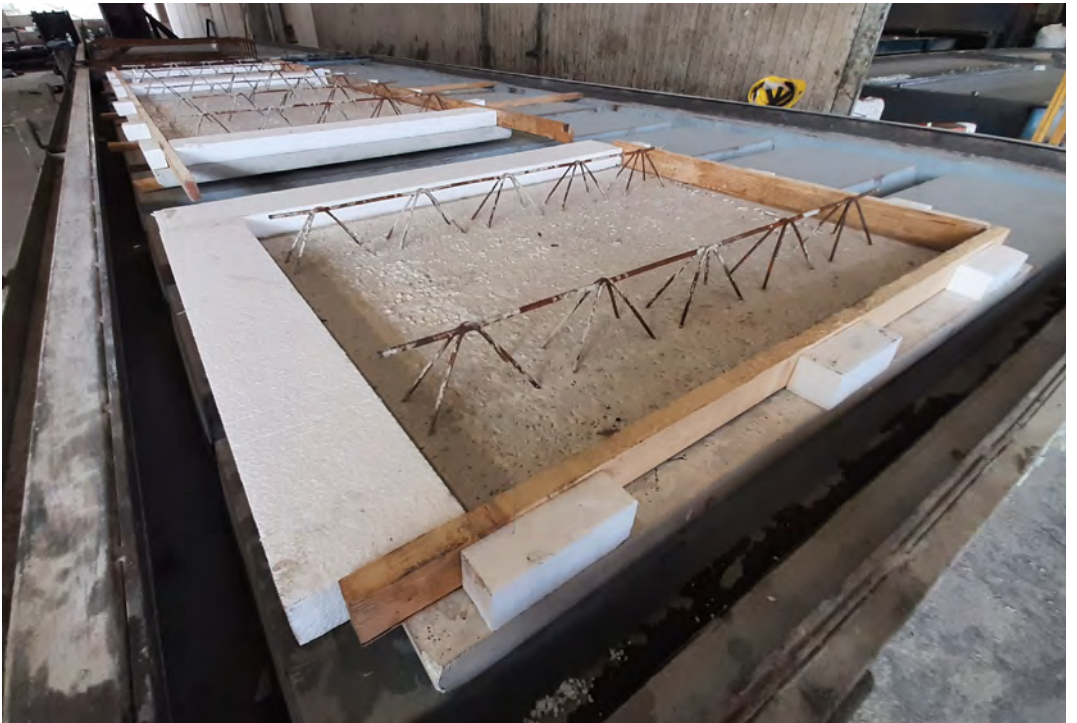
Figure B.18-19: Preparation to the novel lightweight mortar (LWM) casting
