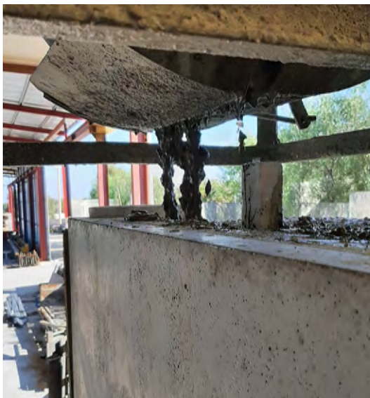
Figure E.47-48-49: LWSC casting through successive layers and with low velocity
