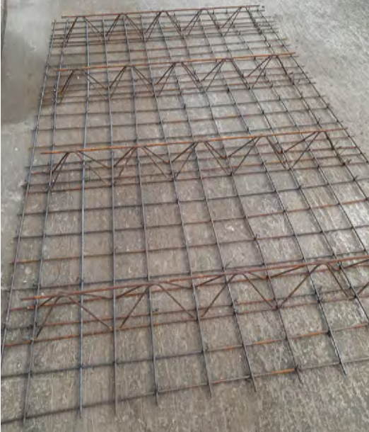
Figure B.1: Labour assembling of the panel reinforcement.
