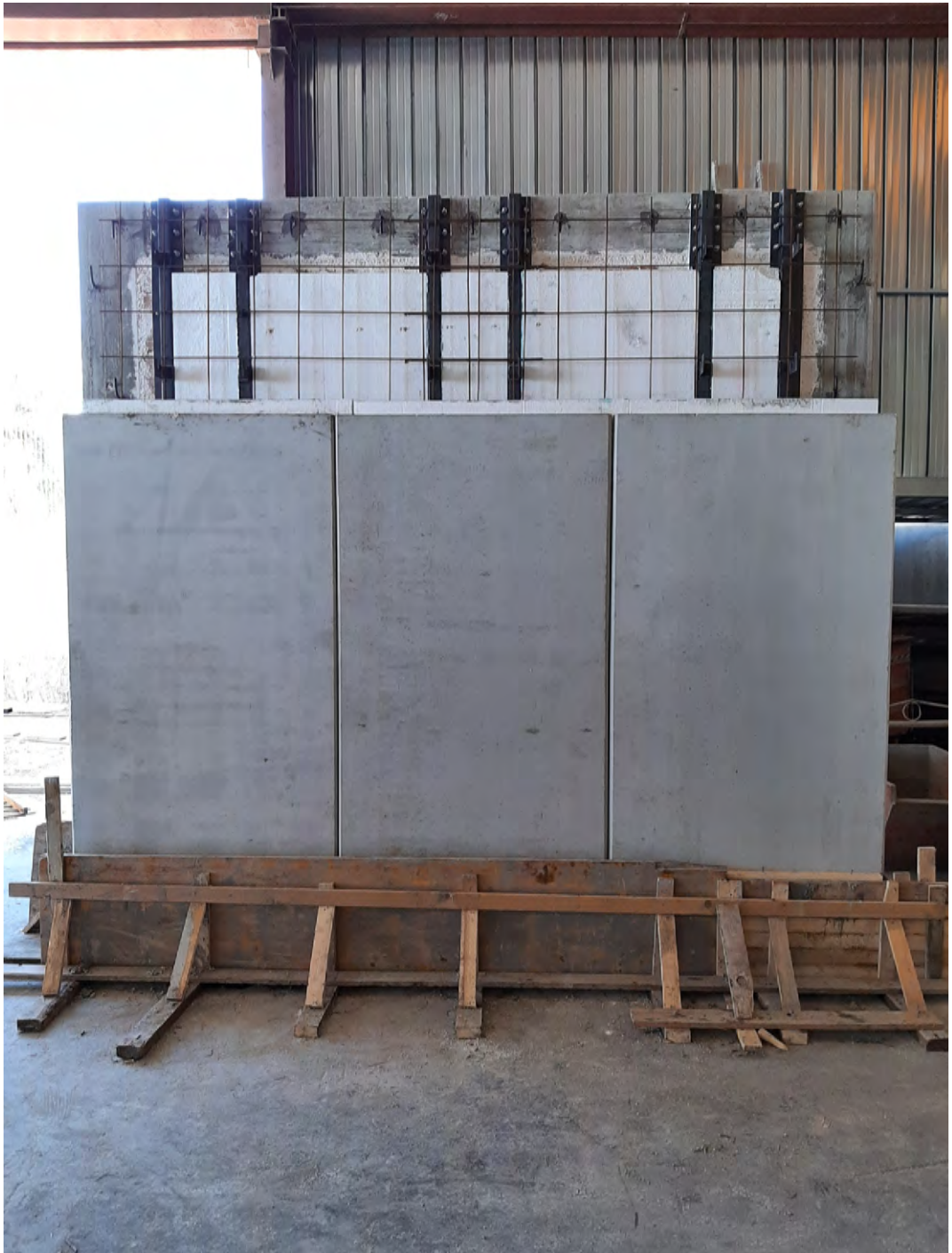
Figure E.32: Coupling the first row of panels with the wall
