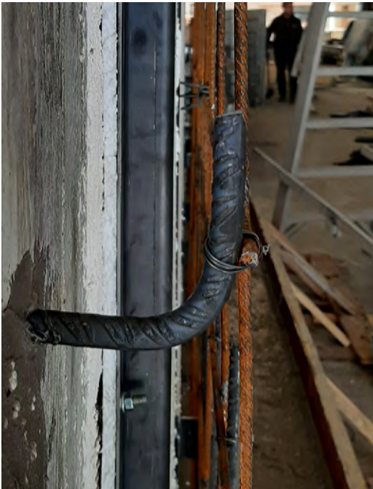
Figure E.24-25: Binding of the post-installed bars with the reinforcement mesh
