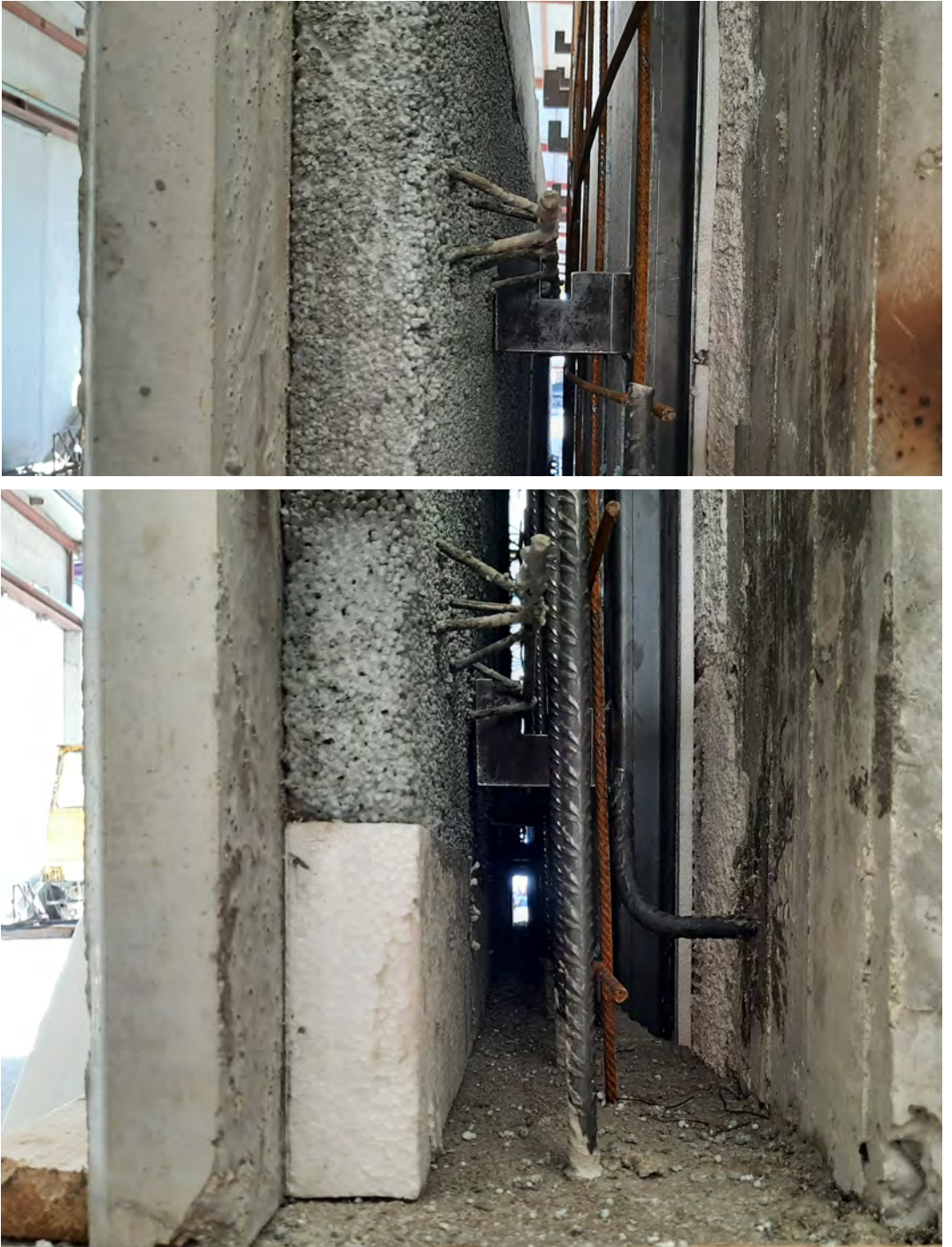
Figure E.33-34: Anchoring details (lateral view): upper and lower connection
