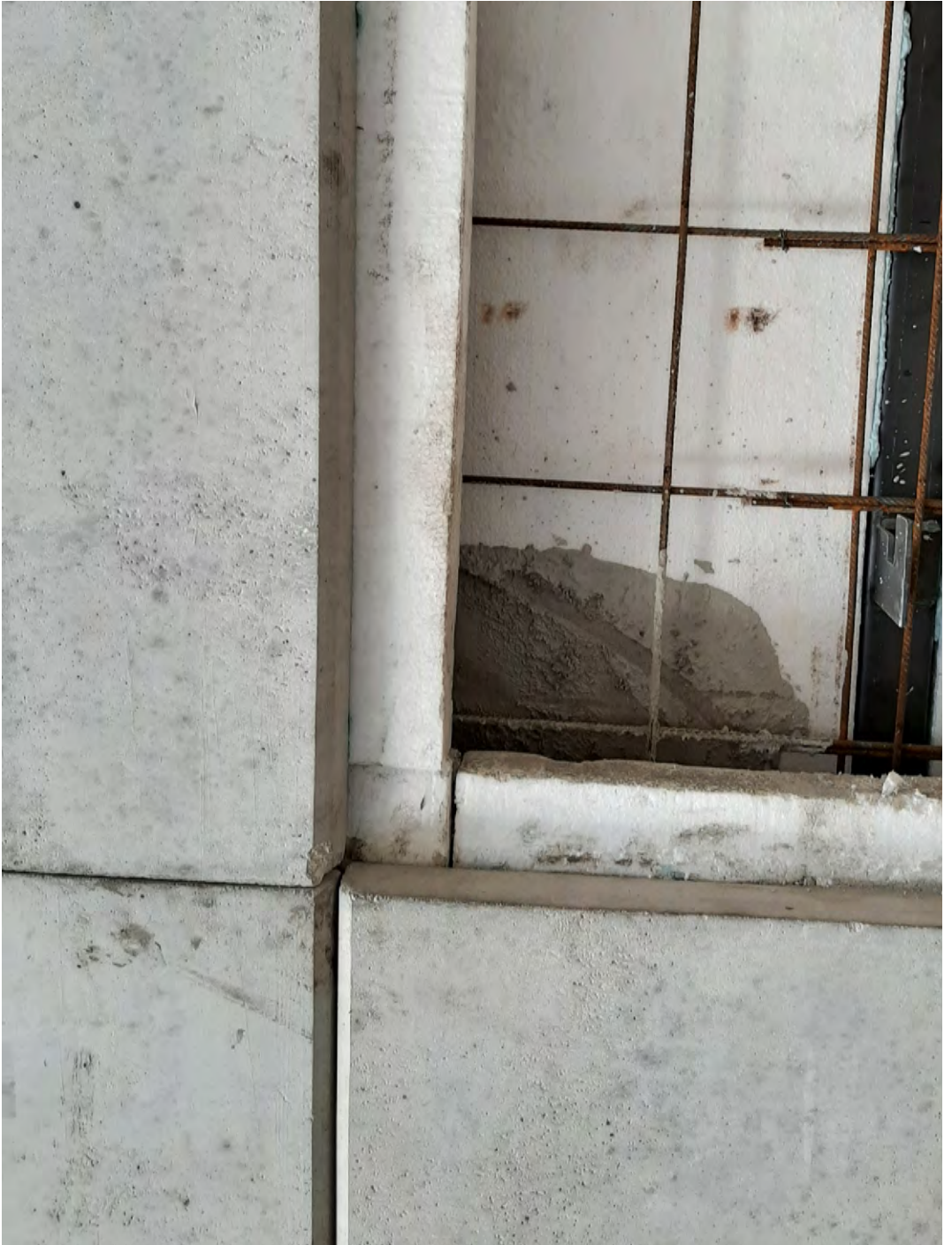
Figure E.42: Detail of junction among the two different rows of modules (front view)
