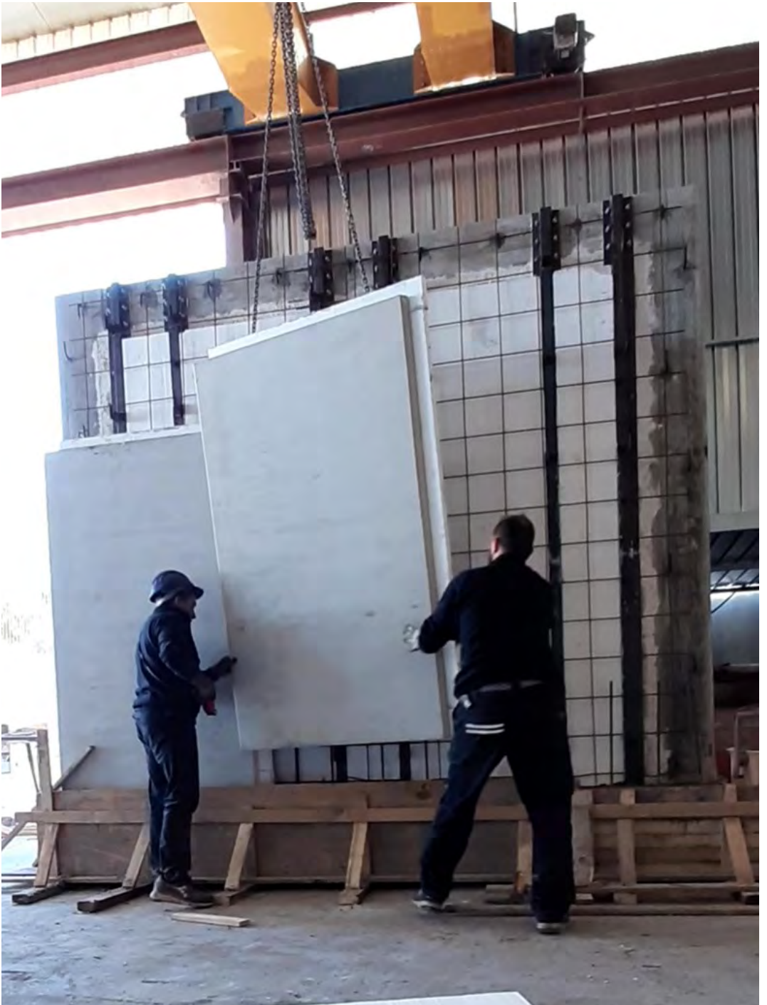
Figure E.31: Installation of the second PC module
