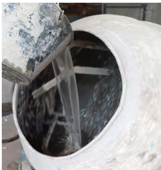
Figure A.7: Addition of water to the premixed compound
