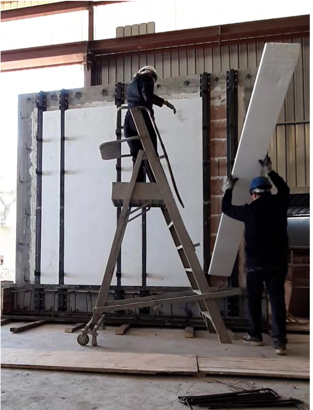
Figure E.18: Gluing of the thermal insulation panels in rEPS
