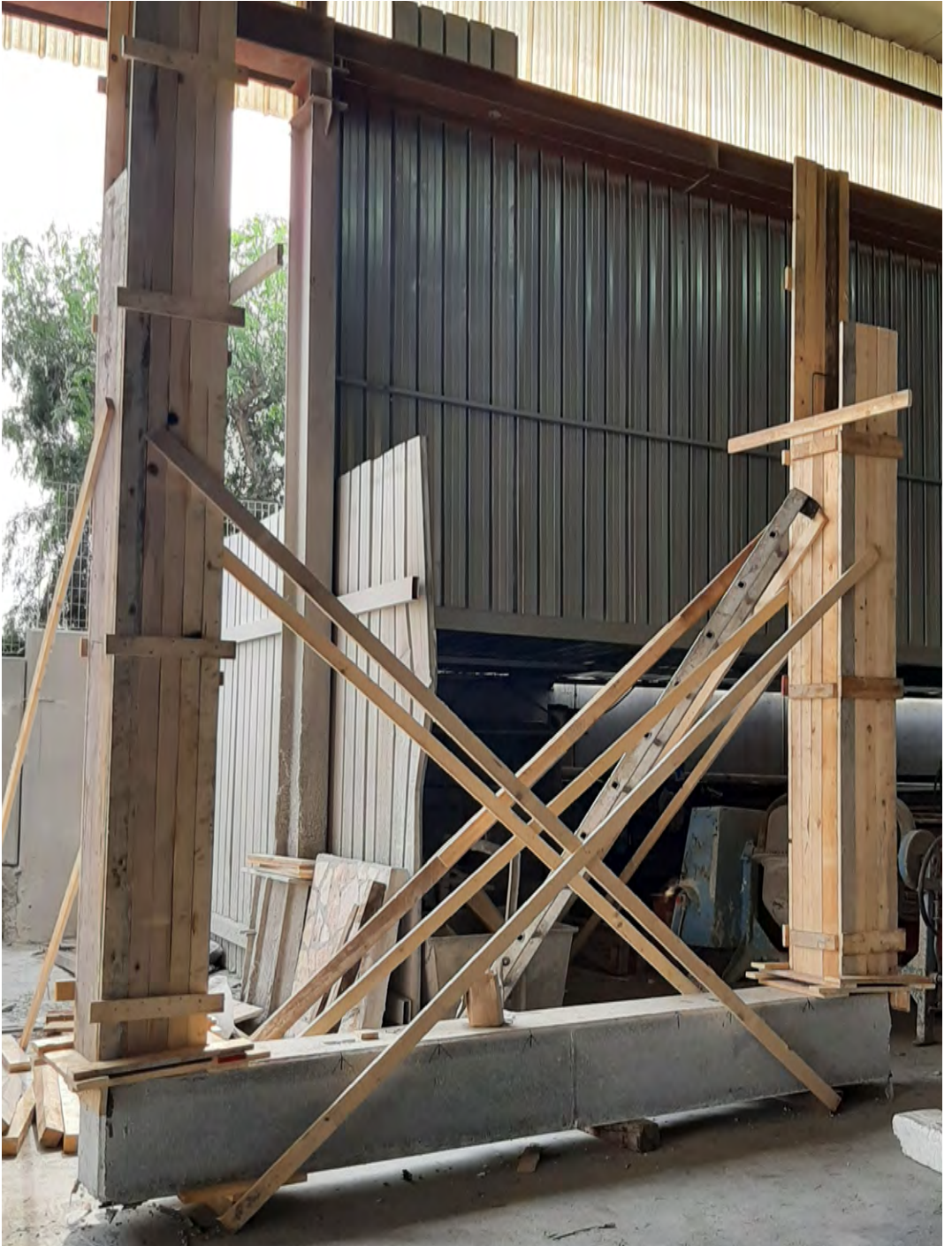
Figure C.2: Construction of the pillars
