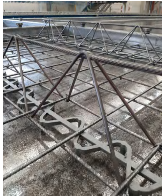
Figure B.2: Placing of the spacers and arrangement of the reinforcement.
