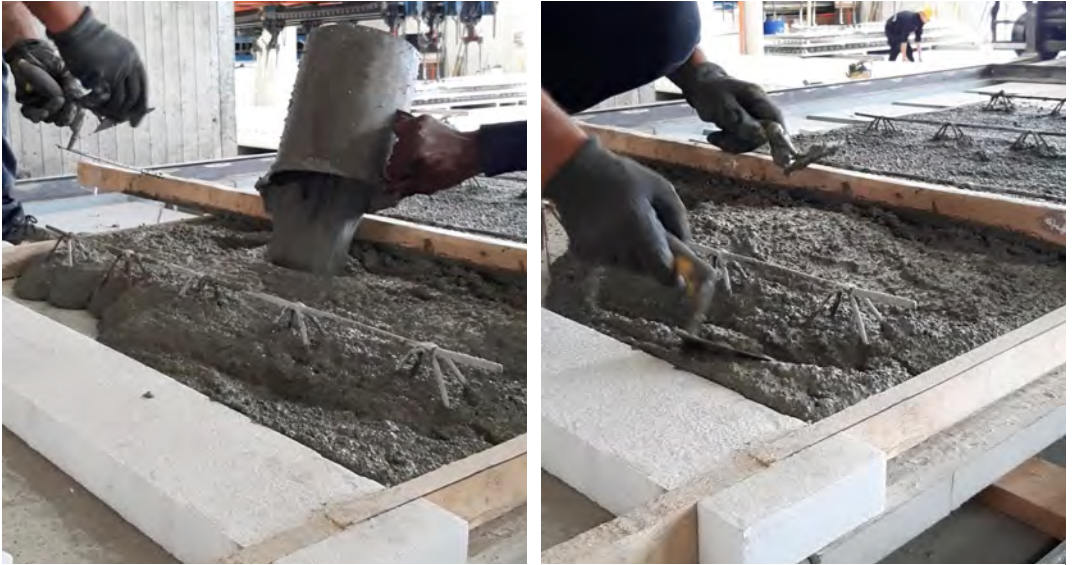
Figure B.21-22: Spreading of the fresh LWM on the inner surface of the base module
