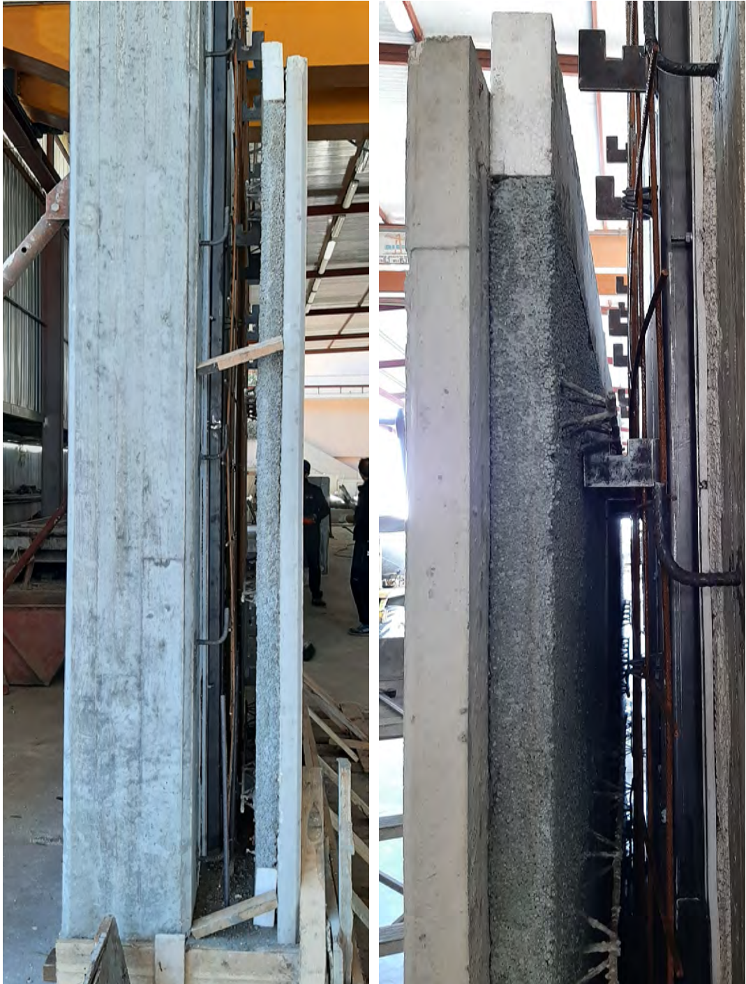
Figure E.29-30: The PC module accousted to the wall: lateral view
