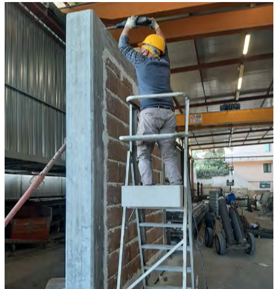
Figure E.1-2-3: Drilling of the concrete frame up to the calculated depth for chemical injection and anchoring of post-installed reinforcing bars and connectors
