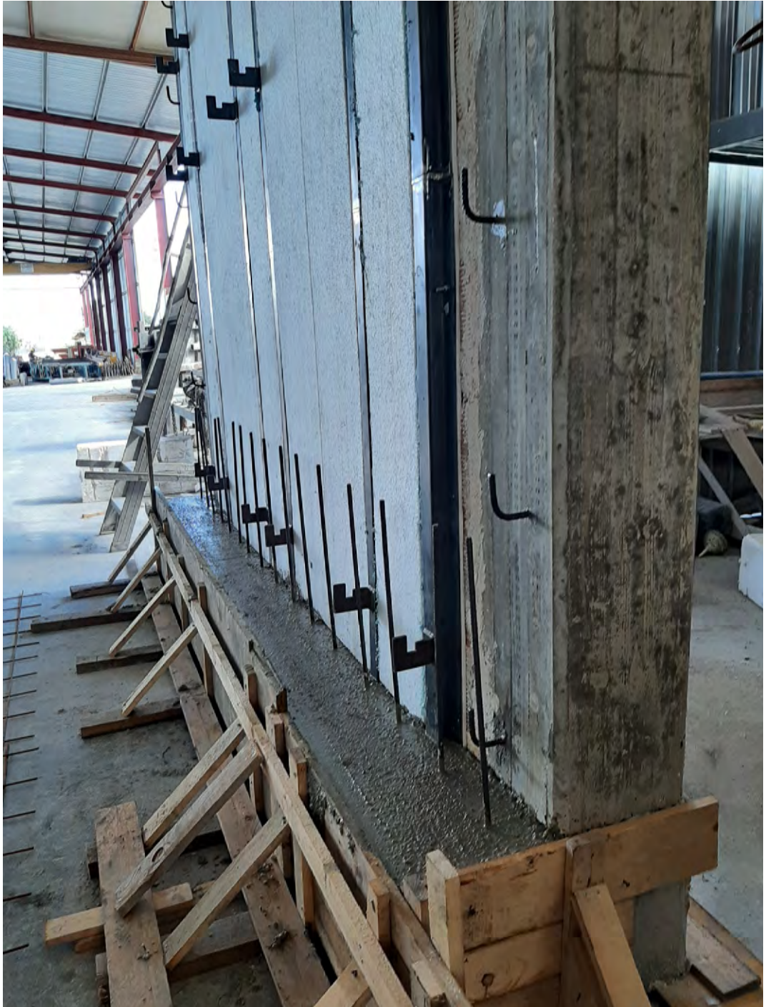
Figure E.21: Concrete casting of the system foundation
