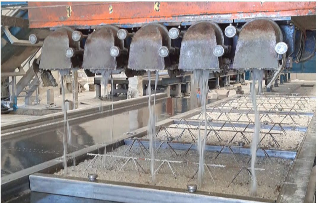
Figure B.11-12: Automatic concrete casting by means of the bridge crane
