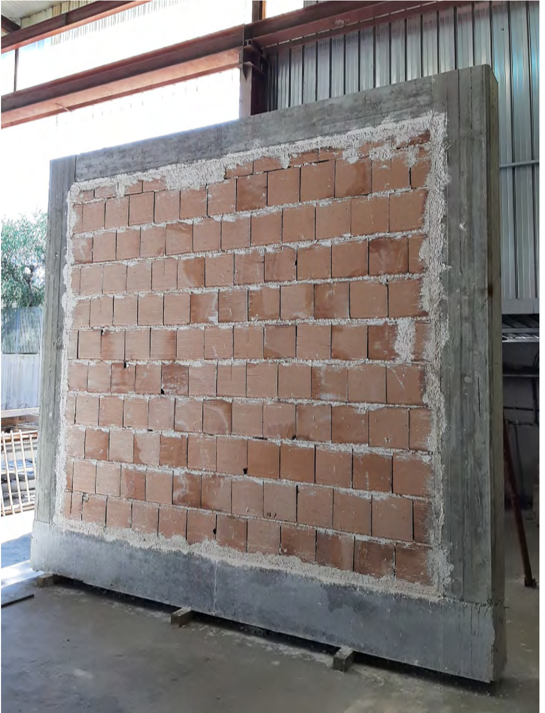
Figure C.4: Concrete frame of the wall sample
