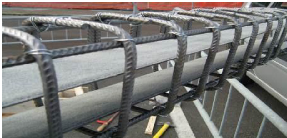
Fig. 7. Realization of the cage for the specimens reinforced with CFRP strips.
