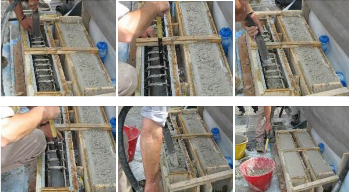
Fig. 8. Constructive phases of the specimens reinforced with CFRP strips.
