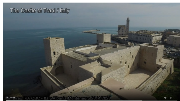
Figure 8. Screenshot, from active “Media” hotspot, showing the inaccessible roofs .
