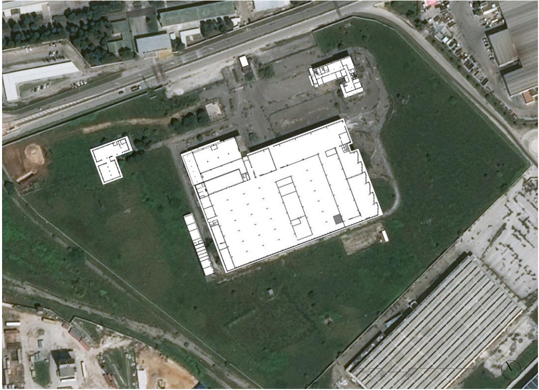
Figure 4.4.2-3 Existing former Radaelli Sud factory morphology.
